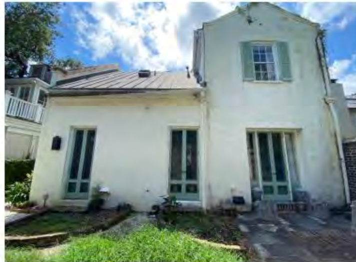
Looking West at rear of Existing House
