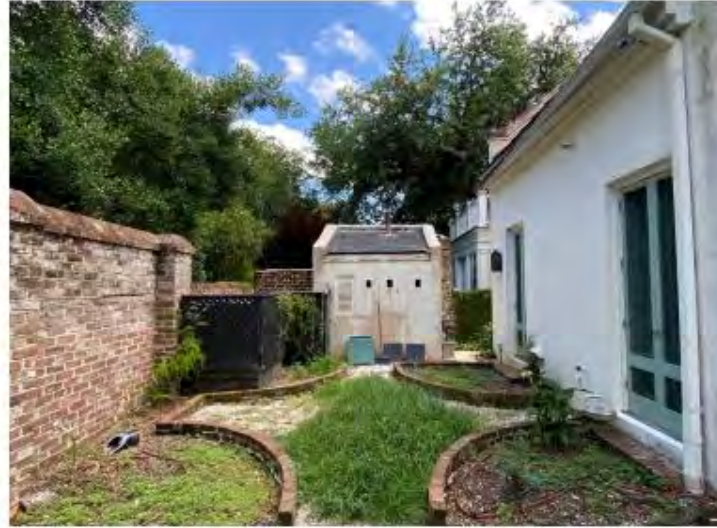
Looking South at Tool Shed
