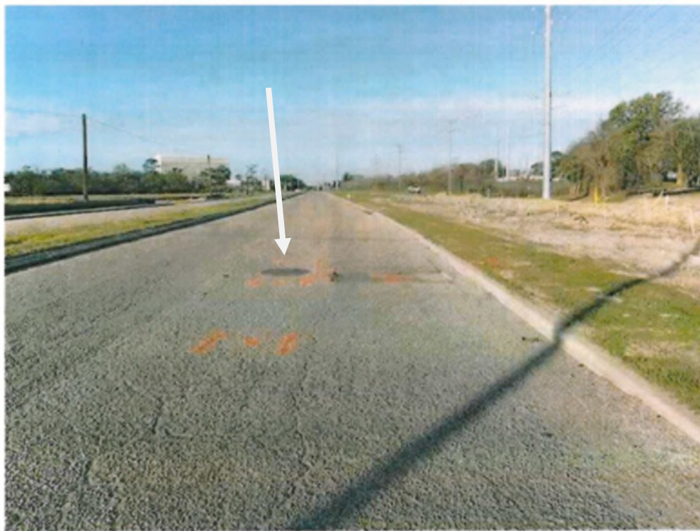
Property of United States Infrastructure Corporation Photo taken on 3/9/2020 8:53:53 AM
