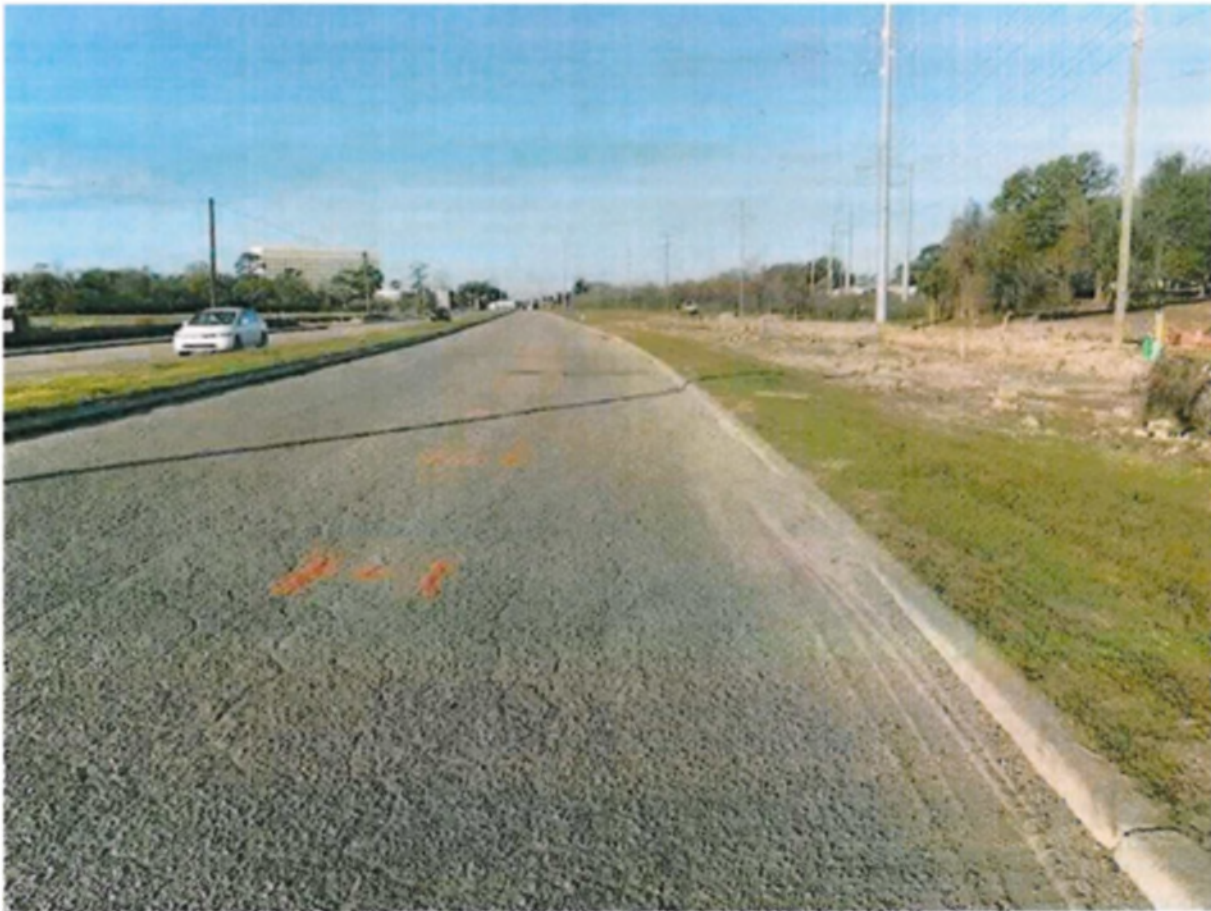
Property of United States Infrastructure Corporation Photo taken on 3/9/2020 8:53:46 AM
