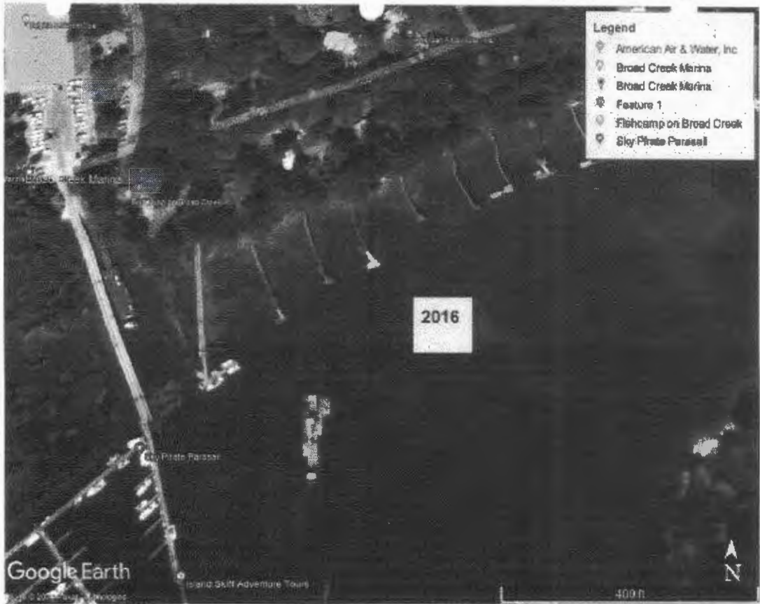
Aerial Image from SFH Exhibit 14 depicting BCM pier, J&W barge, and former SFH dock.
