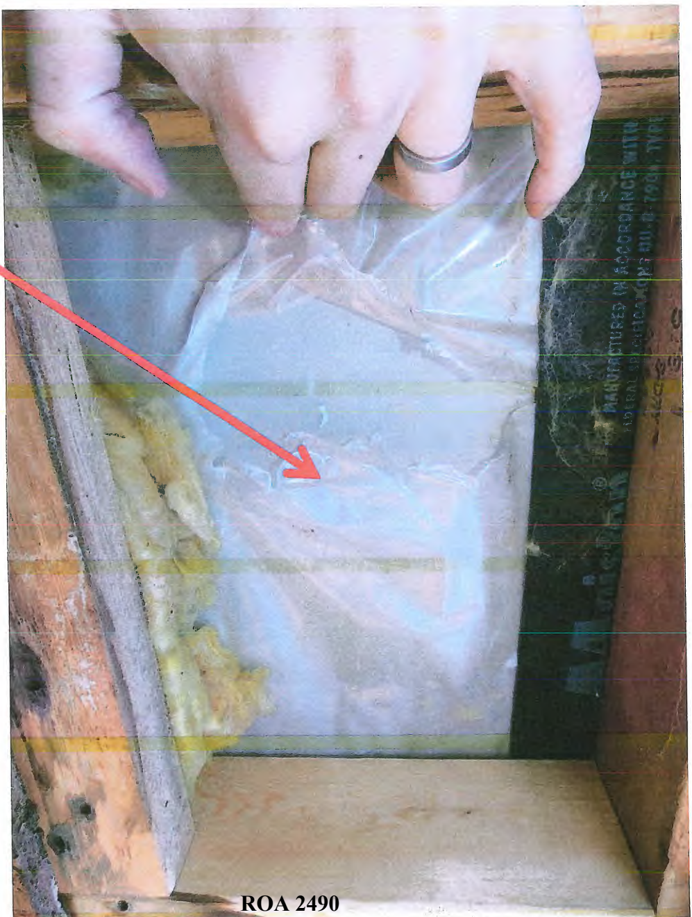
PLASTIC VAPOR BARRIER
