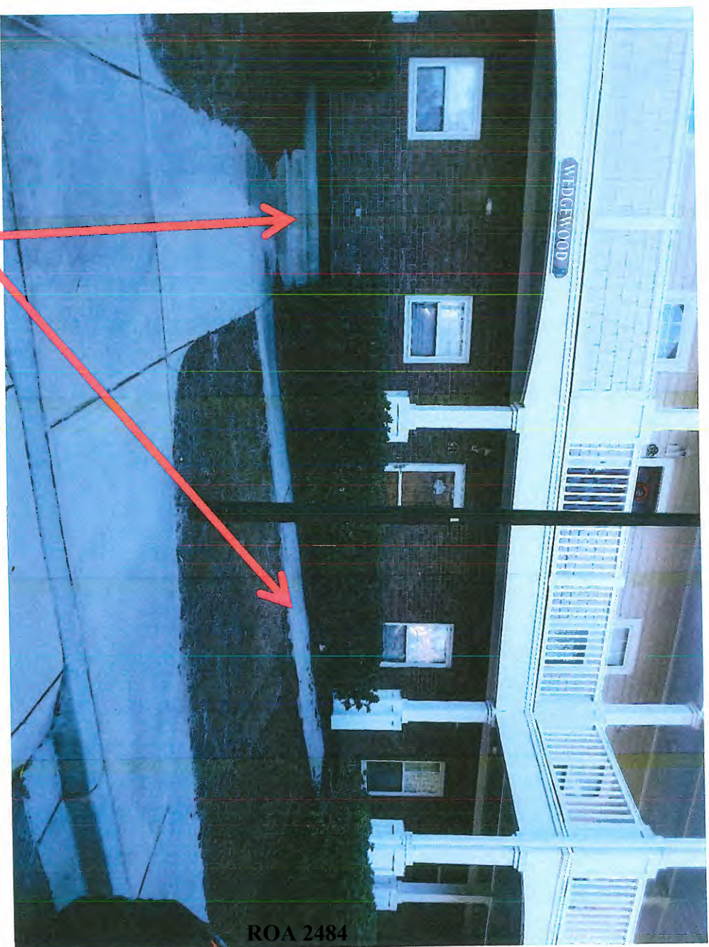
HANDRAILS MISSING
