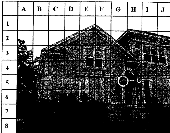
KICKOUT FLASHING IN PLACE
