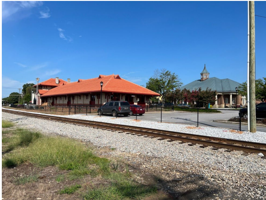
Figure 1 (showing Appellant's fence relative to the Depot building, the east [public] parking lot, and CSXT right of way)
