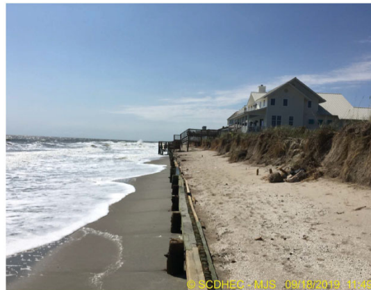
Illustration 7 Bulkhead and High Tide Line
