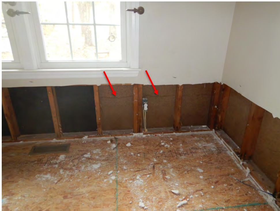
Photo 13 – Interior conditions at the subject residence with the waterline stain indicated. Photo by ABS taken 12/13/2018.
