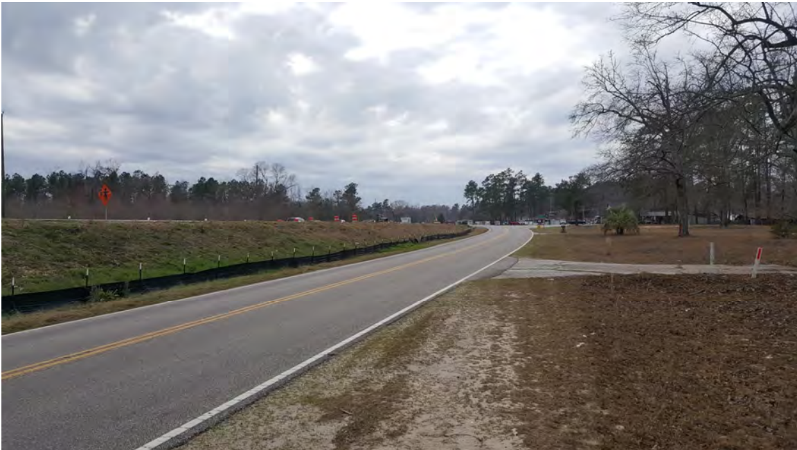
Photo 7 – This photo taken during construction depicts the new roadbed substantially higher than the existing road in front of the Marlowe property, looking west. Photo provided by Hopkins Law Firm.
