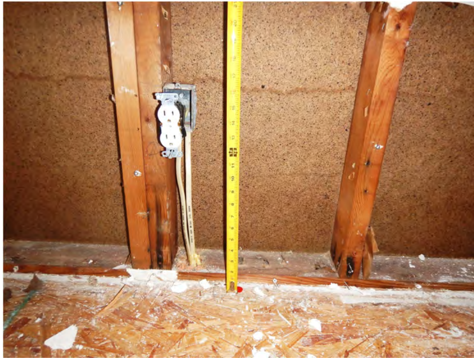
Photo 14 – Waterline stain mark on the inside of the fiber board exterior wall sheathing at approximately 16- to 17-inches above the subfloor. Photo by ABS taken 12/13/2018.
