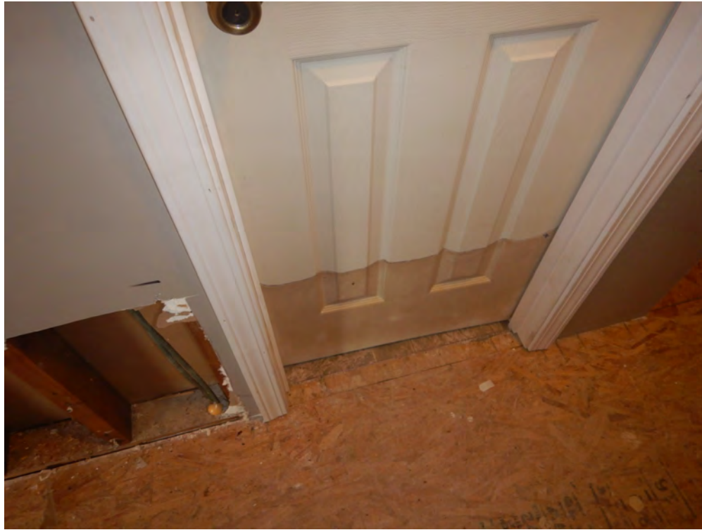
Photo 12 – Water stain mark on an interior door panel. Photo by ABS taken 12/13/2018.
