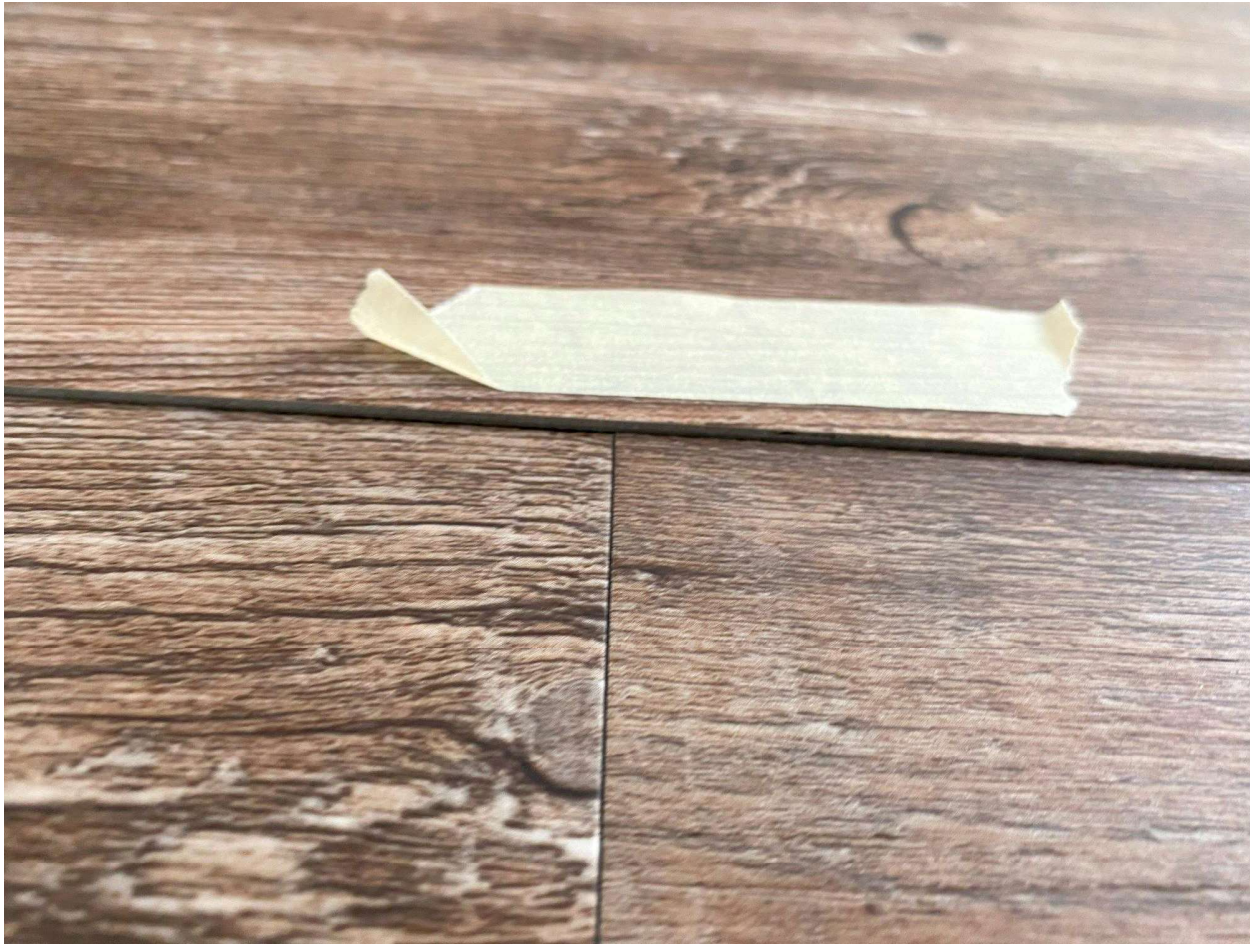
Picture 5: Lifting and peeling planks
