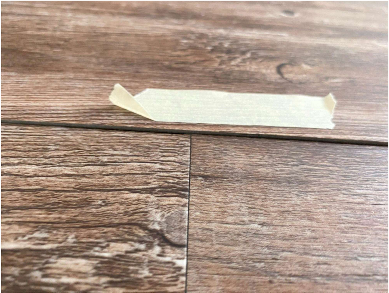
Picture 5: Lifting and peeling planks
