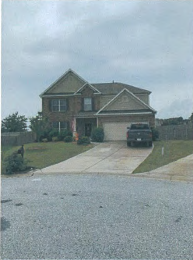
11 Chatham Court Two story
