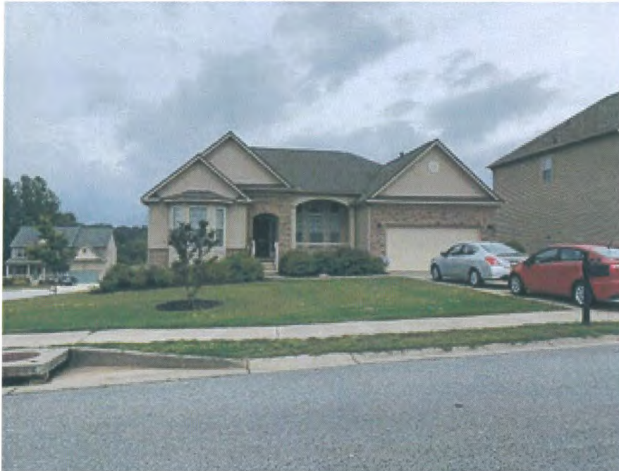
305 Amesbury One story with roof over garage
