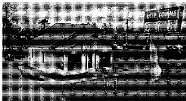
This building does not meet Standard j.
