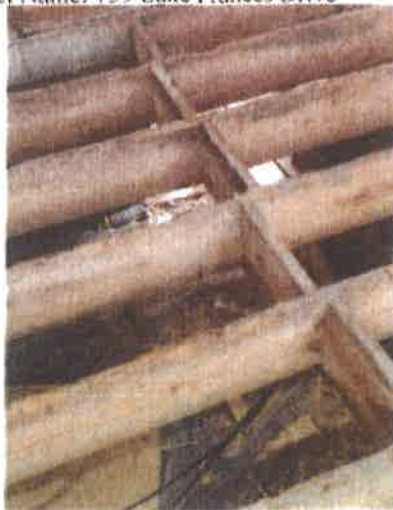
Photo 17. Deteriorated 2x10 floor joists (typical).
