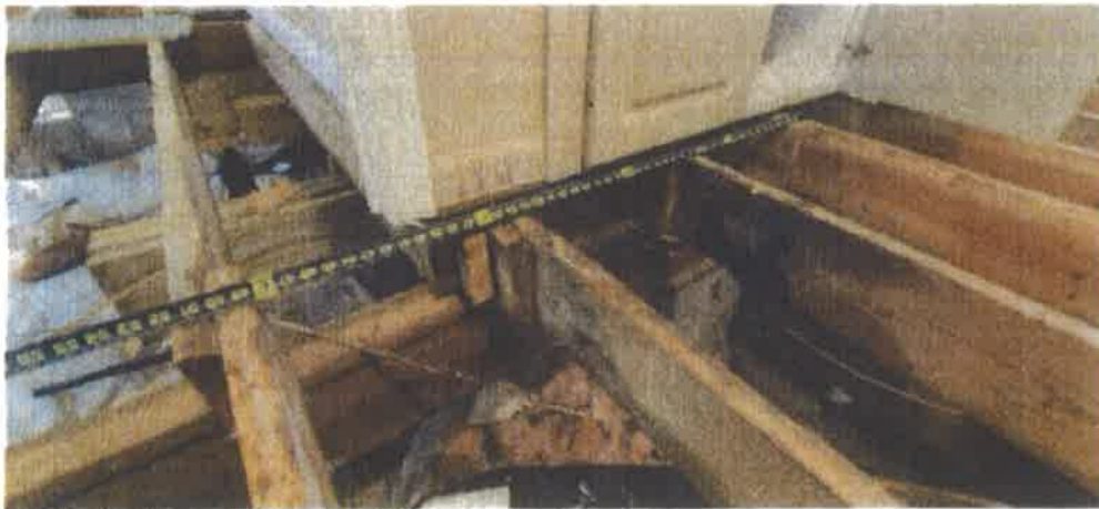
Photo 24. Drop girder in kitchen area.
