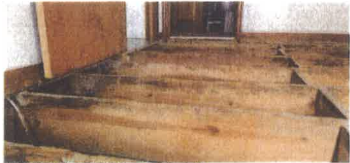
Photo 17. Deteriorated 2x10 floor joists (typical).
