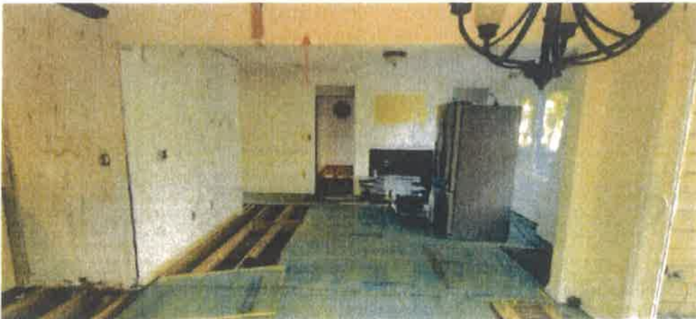
Photo 8. Second floor drop girder over dining area (red arrow).
