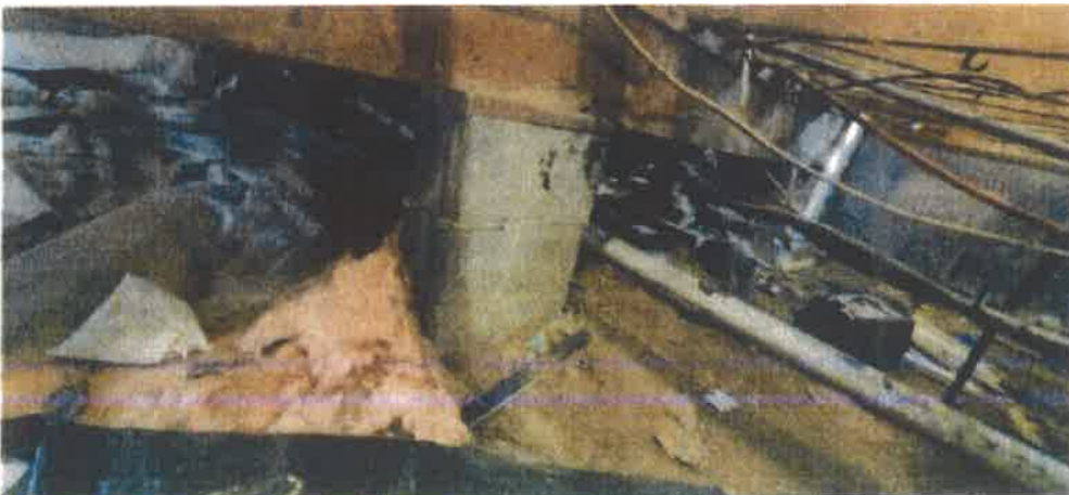
Photo 25. Drop girder under kitchen area.
