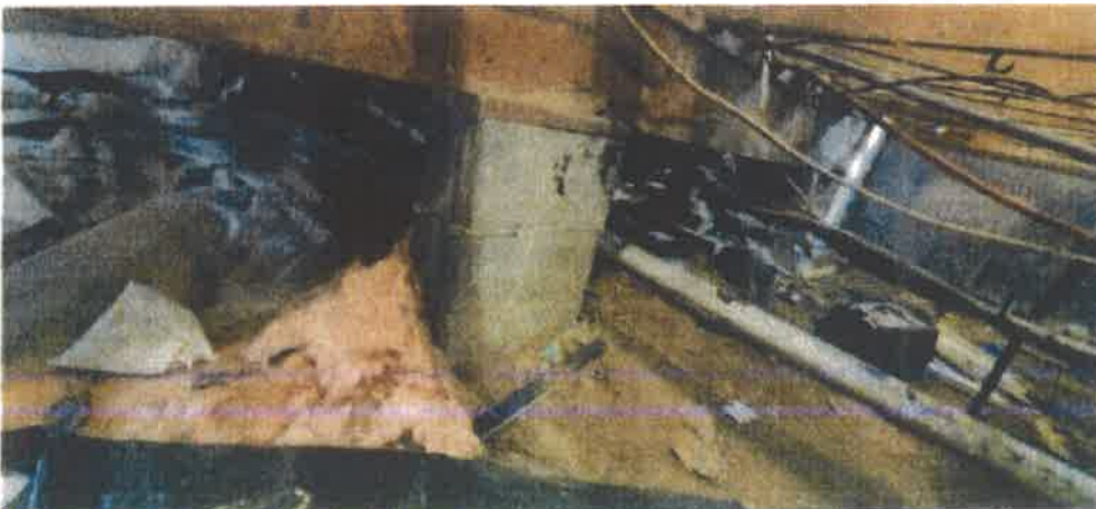
Photo 25. Drop girder under kitchen area.
