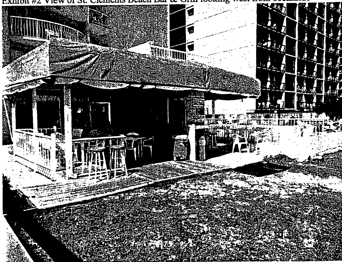
Exhibit #2 View of St. Clements Beach Bar & Grill looking west from oceanside
