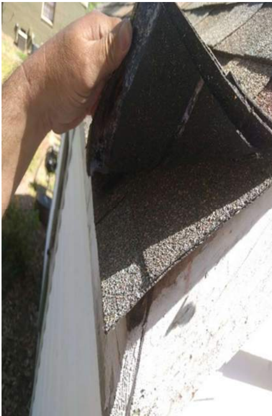
NO STARTER USED ON SHED
