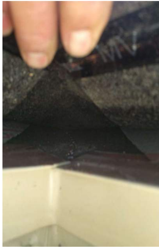
NO VALLEY TREATMENT OR FLASHING
