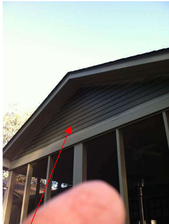
Existing Screen Porch Siding With A 4" Exposure
