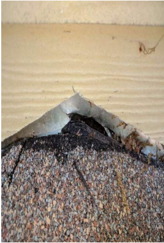
CUT FLASHING
