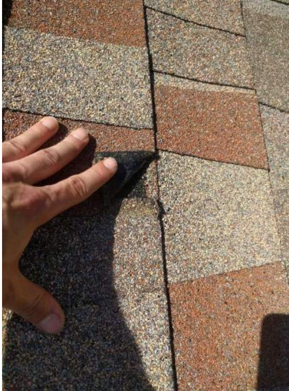
OVERLAPPED SHINGLES
