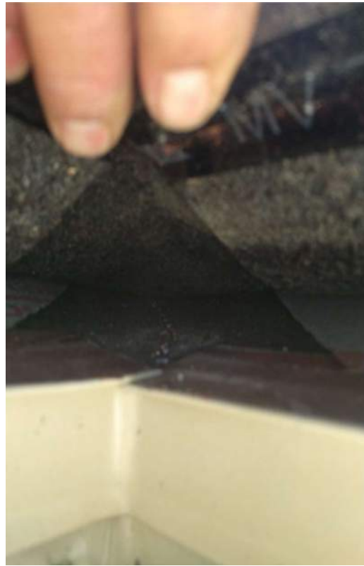
NO VALLEY TREATMENT OR FLASHING
