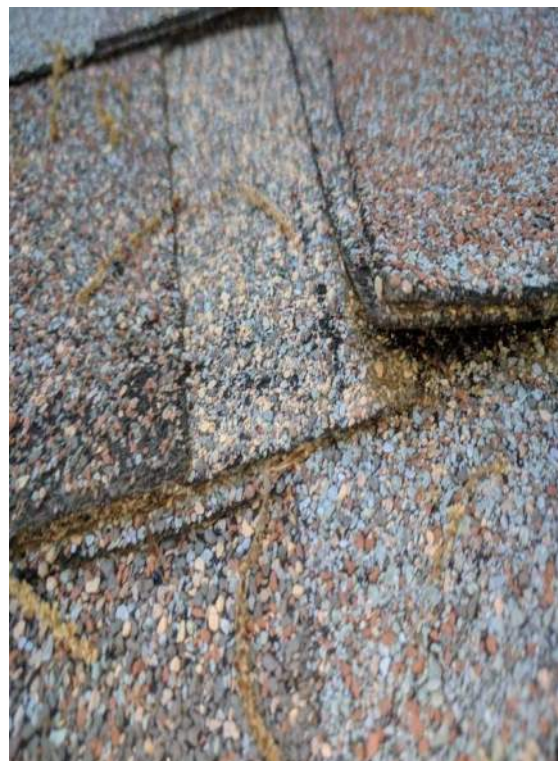
OVERLAPPED SHINGLES
