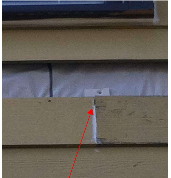
NO NAILS IN BUTT JOINT
