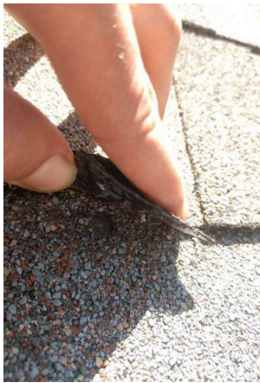
OVERLAPPED SHINGLES
