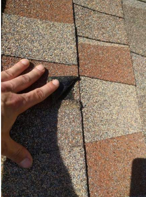
OVERLAPPED SHINGLES
