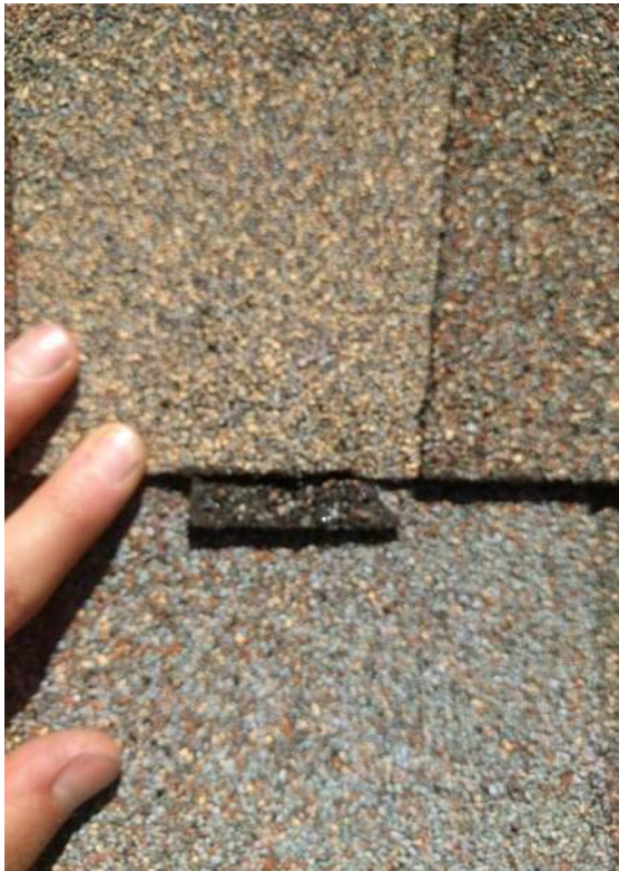
LOW NAILS INSTALLED WITH SKIRT TO COVER
