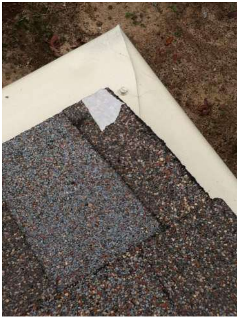
Small Piece Of Shingle Taped On
