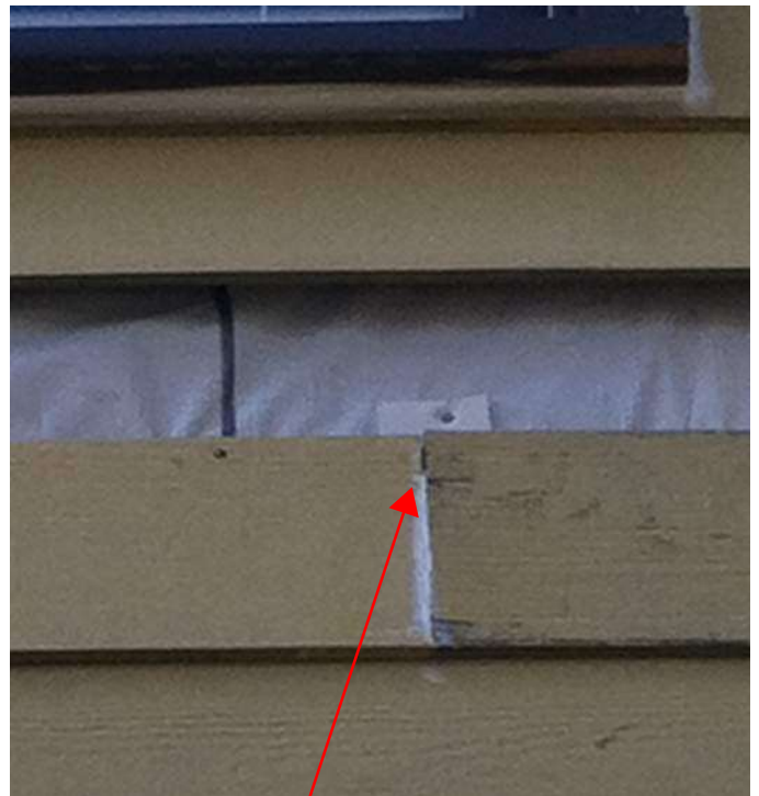
NO NAILS IN BUTT JOINT
