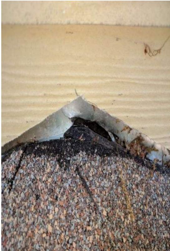
CUT FLASHING
