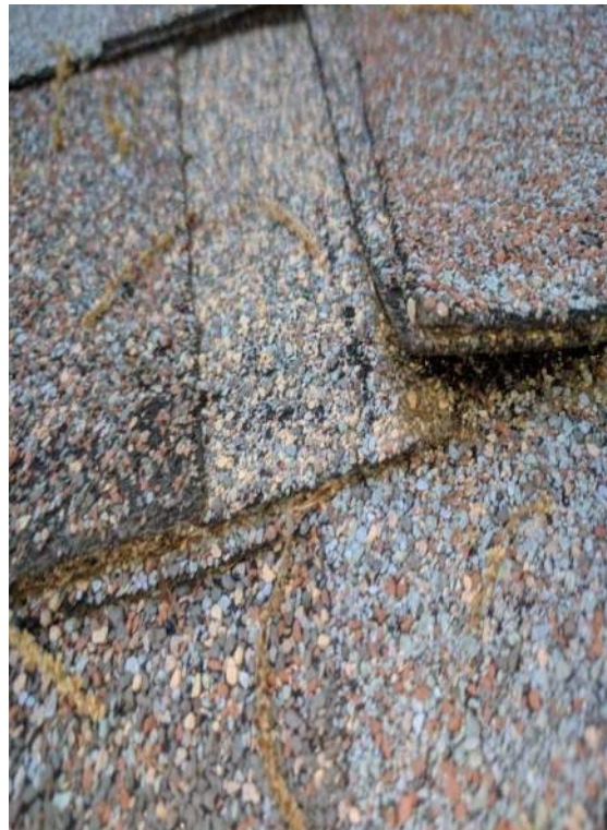
OVERLAPPED SHINGLES
