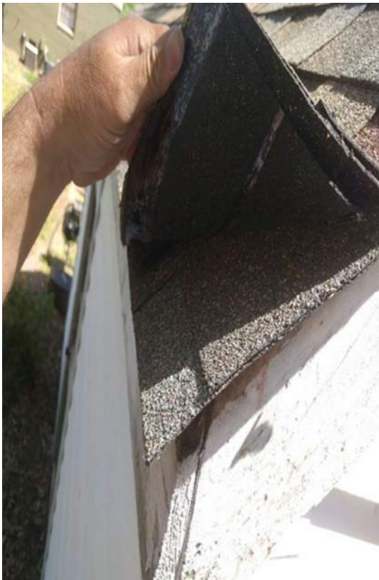
NO STARTER USED ON SHED
