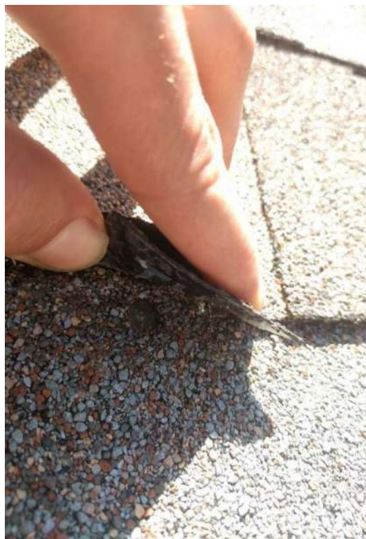
OVERLAPPED SHINGLES
