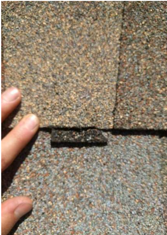
LOW NAILS INSTALLED WITH SKIRT TO COVER
