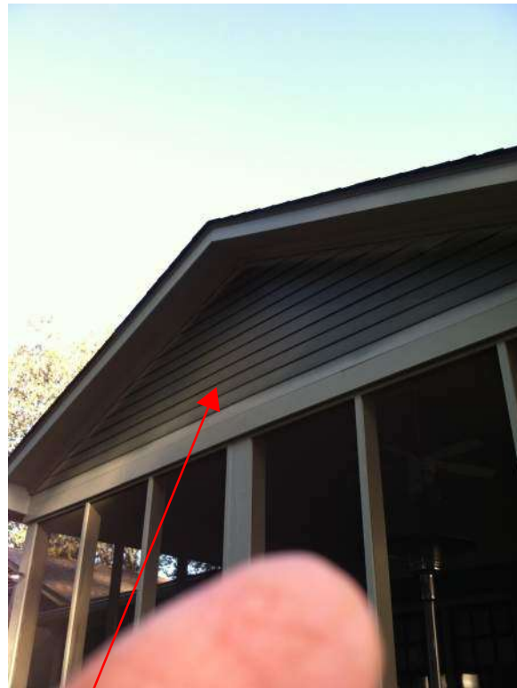
Existing Screen Porch Siding With A 4" Exposure
