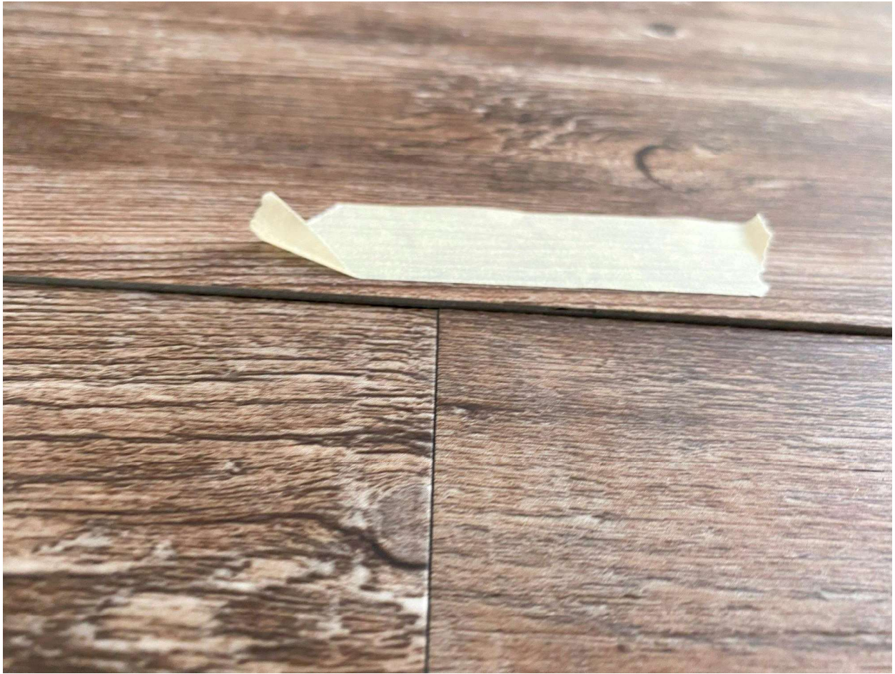
Picture 5: Lifting and peeling planks
