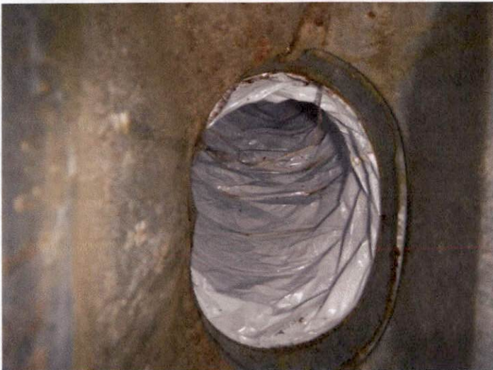
Water at HVAC supply vent.
