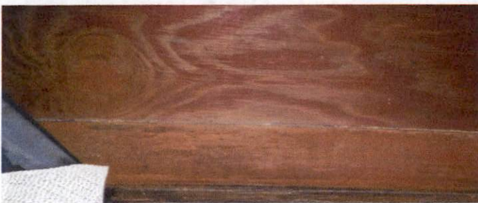
Very heavy water damage at kitchen sink cabinet. Organic growth likely.
