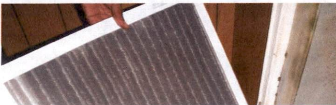
Heavy rust at supply vent due to too much humidity being emitted by HVA intended. Vent boot not connected at floor enabling exterior air into conditi visible damage.
