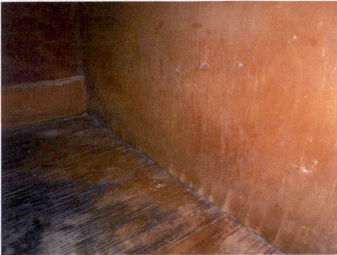
Very heavy water damage at kitchen sink cabinet. Organic growth likely.
