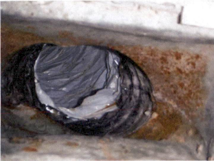
Heavy rust at boot. Old and new vent not connected securely enabling craw space.
