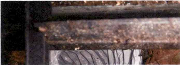
Heavy rust at boot. Old and new vent not connected securely enabling craw space.
