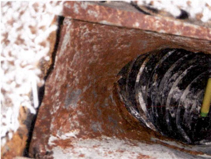
Heavy rust at supply vent due to too much humidity being emitted by HVA intended. Vent boot not connected at floor enabling exterior air into conditi visible damage.
