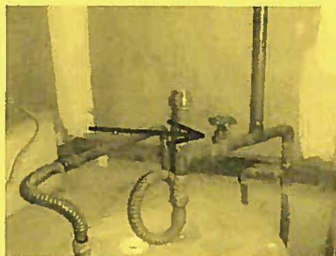
Valve at top of water heater is leaking
