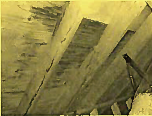
Dry stains in attic, possibly old, confirm all leaks have been repaired
