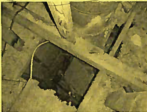
Rust on fireplace box and flue from previous leaks. Open area (chase) around fireplace is not sealed
