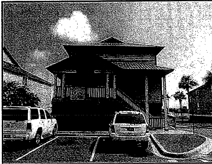
Front of building – Unit 1-A on the first habitable floor
