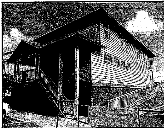
Another view of the front and west side of the building. Note the stairs on the west are not usable due to rot.
