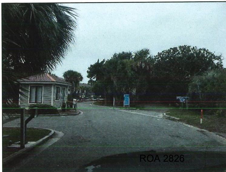
UNIT 1-B MARINERS CAY DRIVE ENTRY GATE
