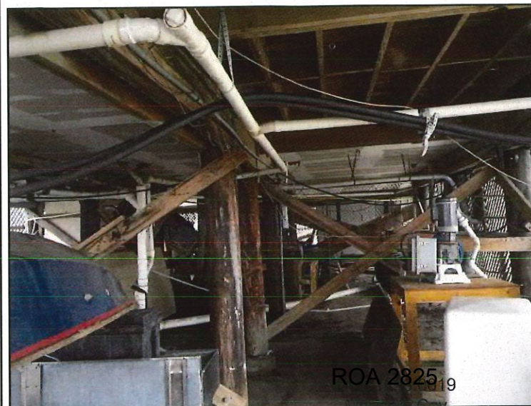
UNIT 1-B MARINERS CAY DRIVE UNDER BUILDING
