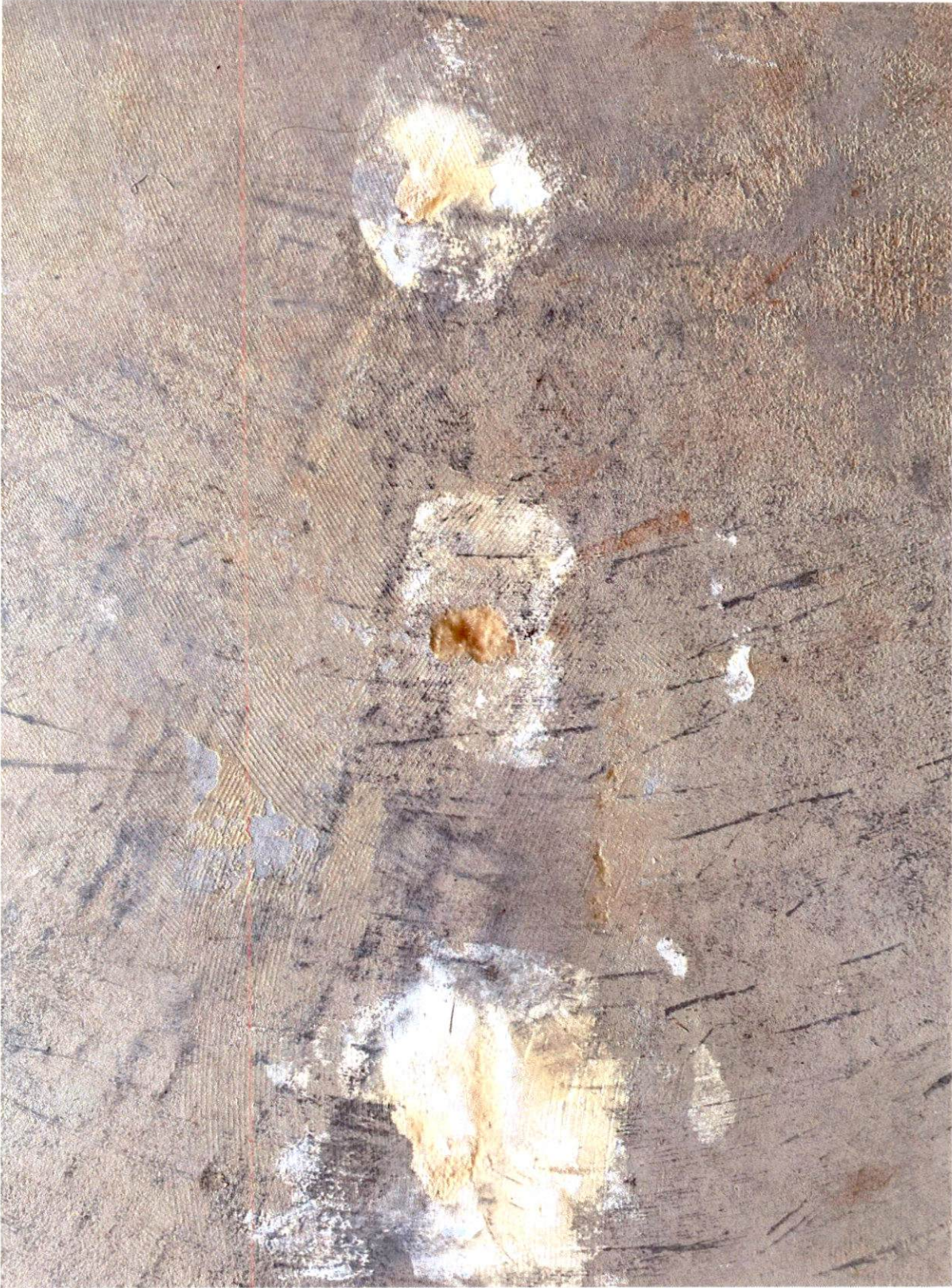
Picture 3: Porous and cracked subfloor absorbed glue
