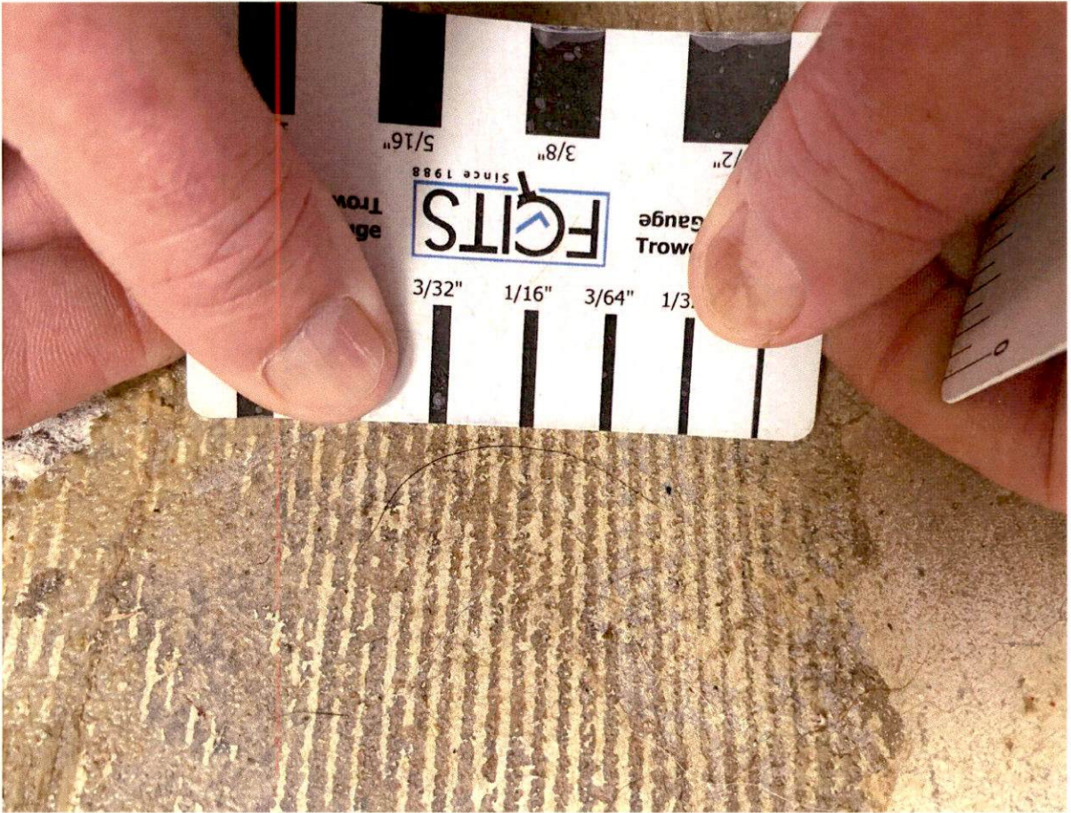
Picture 31: The old installation: 1/16" x 1/16" trowel
