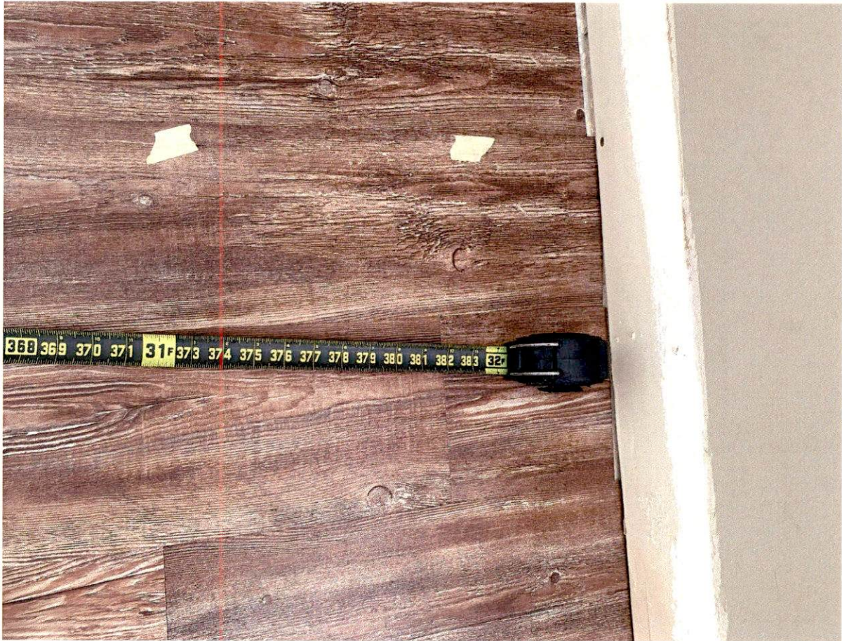
Picture 4: Lifting and peeling planks
