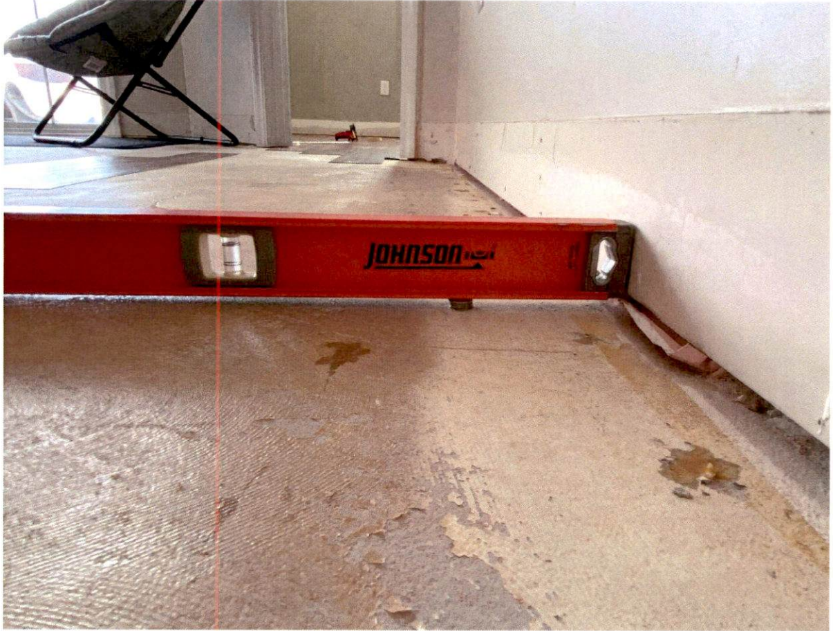
Picture 29: Sub-floor not prepped: major deviations not filled, old paint not removed
