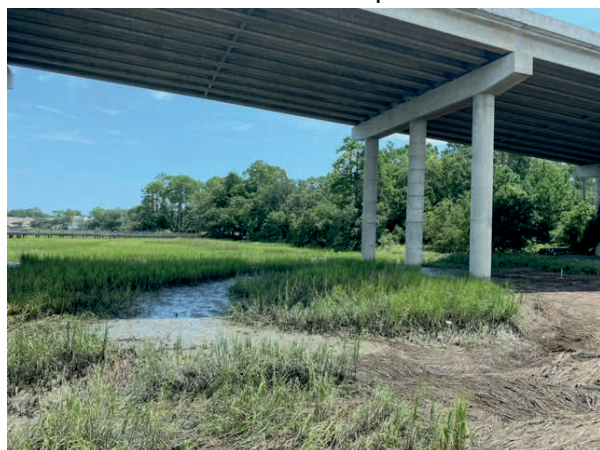
View of subject from public boat landing
