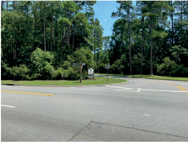
View of subject from Helmsman Way
