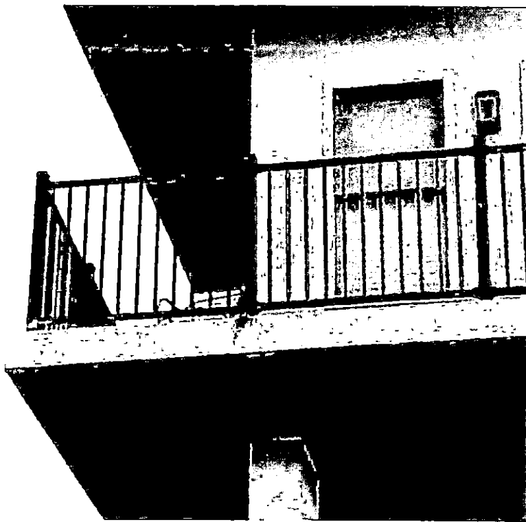
Photos 9 & 10: Corrosion was visible along the outboard edge of the concrete balconies and courtyard terrace in proximity to guardrail post base attachments.
