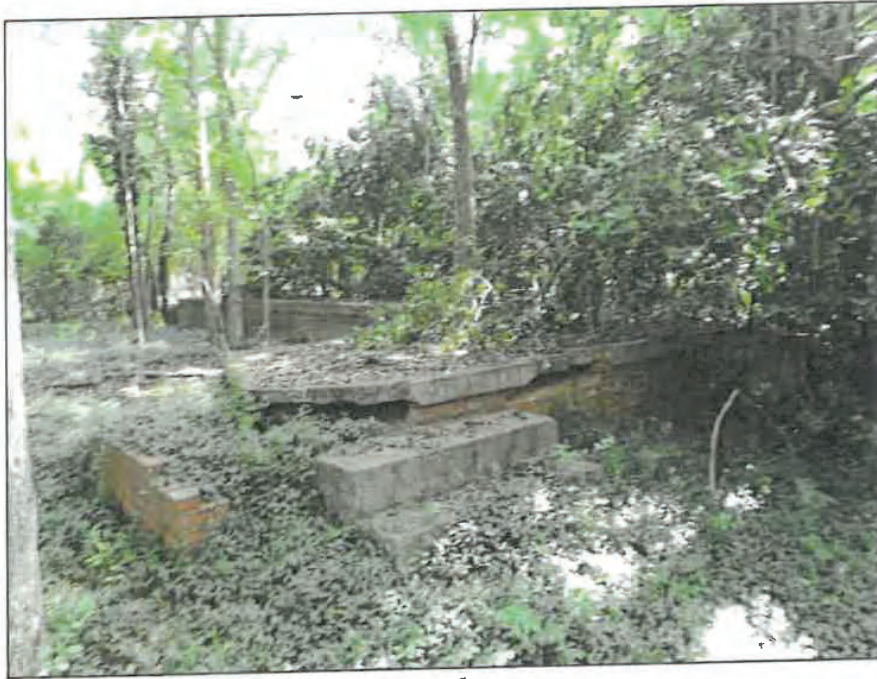
Figure 9. Foundation of the main house, facing southeast.
