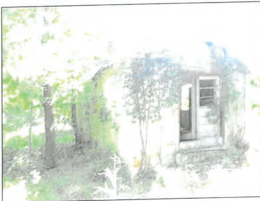
Figure 10. One of the standing outbuildings, facing east.
