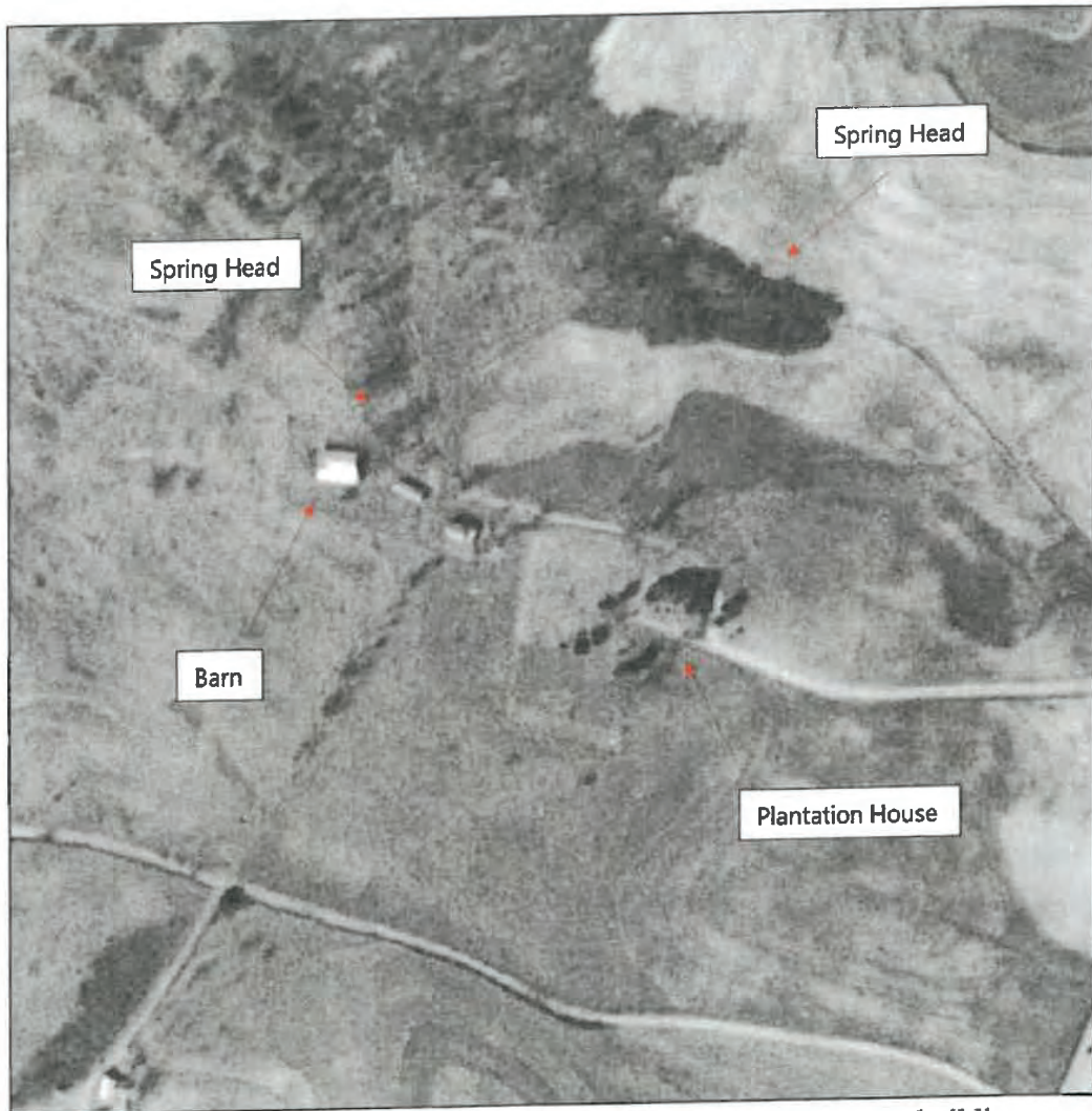
Figure 7. Aerial imagery from 1947 showing Rivoli Plantation, barn, and two outbuildings.
