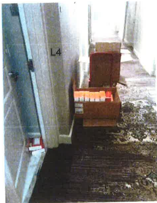
Owner LV Contractor working in L 4 Rooms Door Propped open
