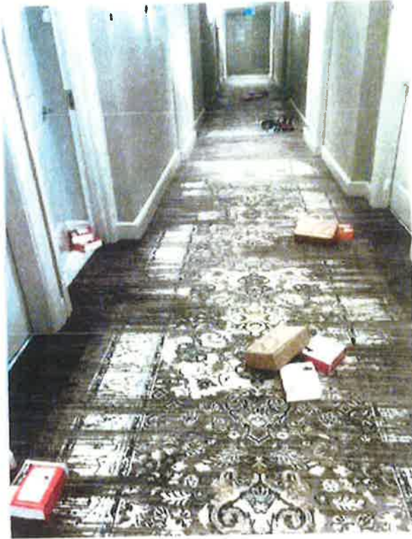
Owner LV Contractor Trash in hallway
