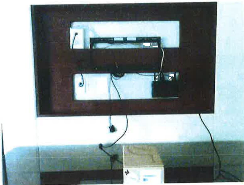
Owner LV installer with stuff on dresser
