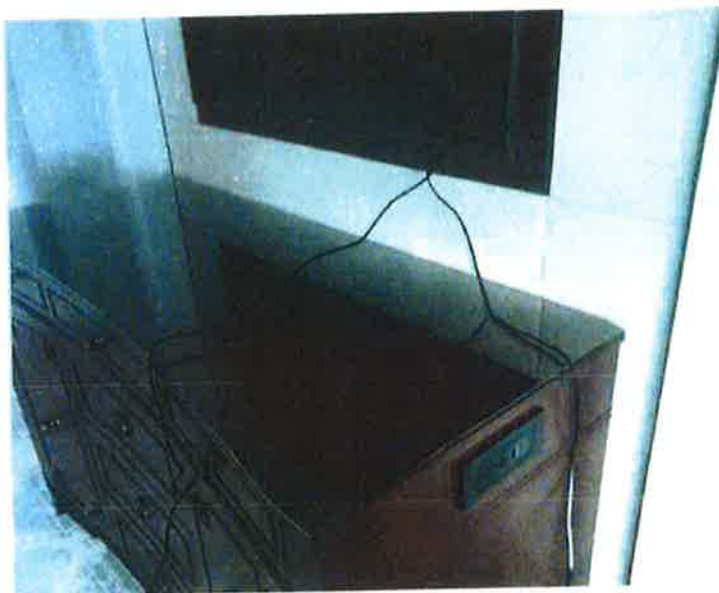
Owner LV Contractor with wire hanging off dresser
