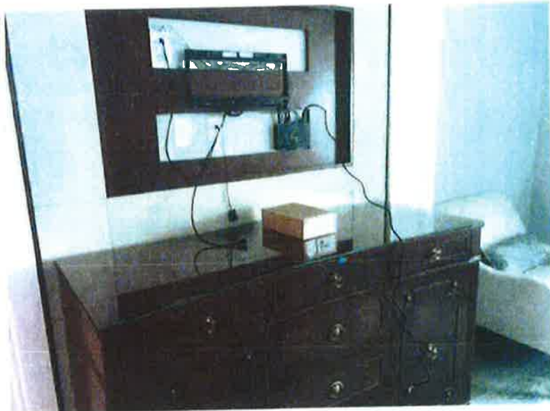
Owner LV Contractor with wire and boxes on dresser
