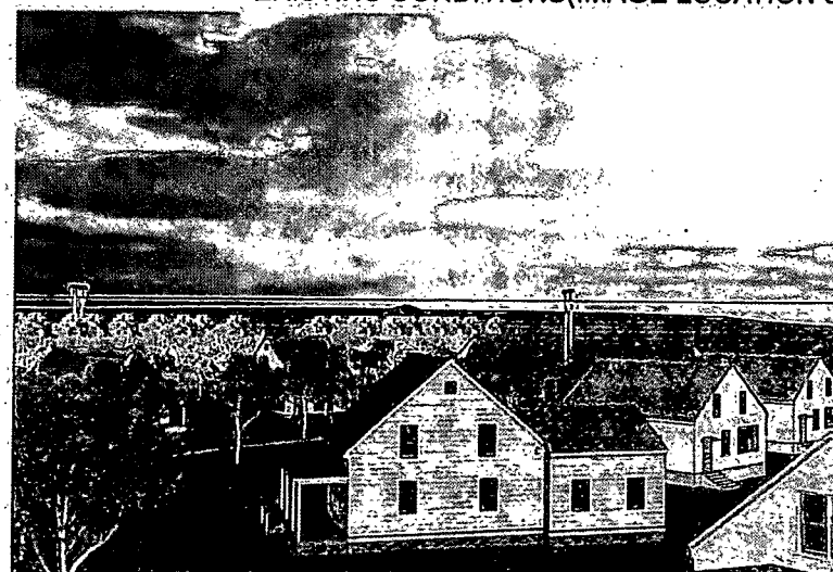
EXISTING CONDITIONS (IMAGE LOCATION 8 30' ABOVE STREET LEVEL)
