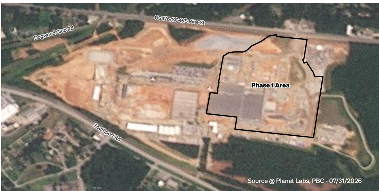
Figure 2 depicts the same boundary on a satellite image from July 2026, which shows large-scale development, tree-cutting, grading, and excavating well outside the Phase I boundary.
