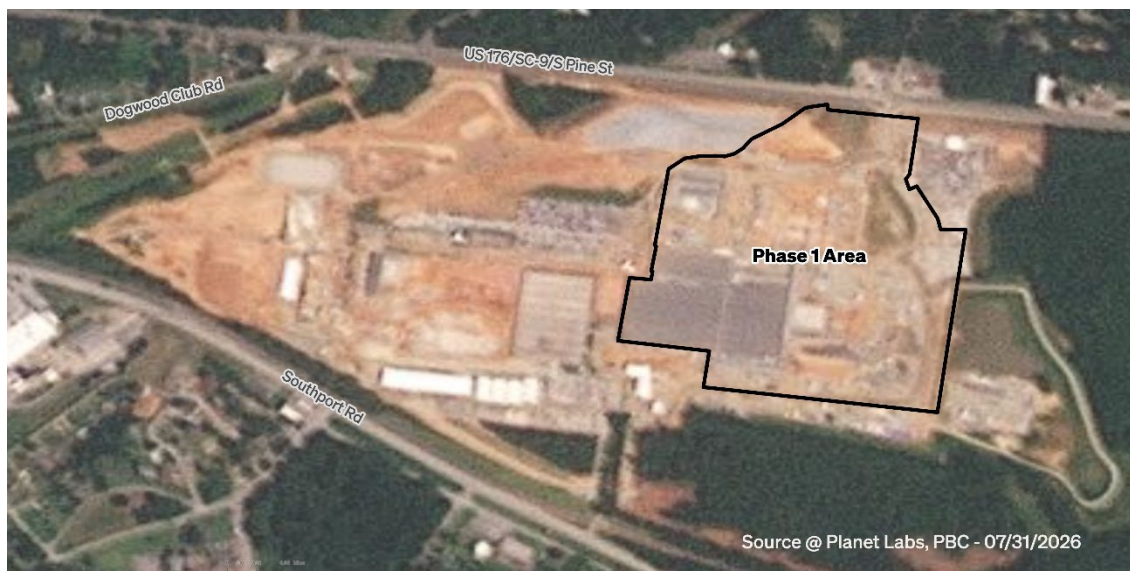
Figure 2 , above, is a satellite image of the site from July 2026 depicting widespread land development well beyond the permitted boundary and footprint of the old Kohler plant.
