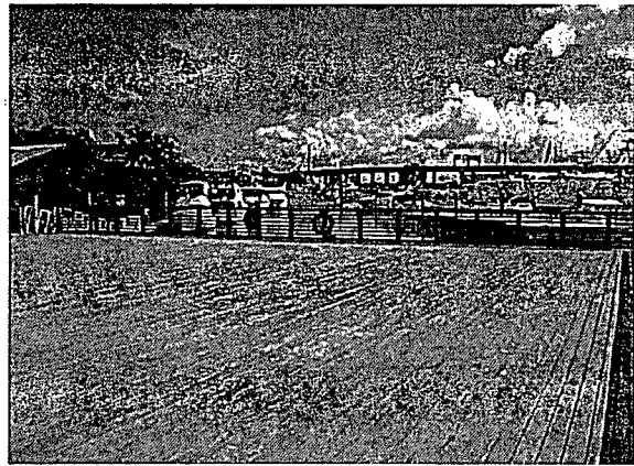
View of Main Deck Area
