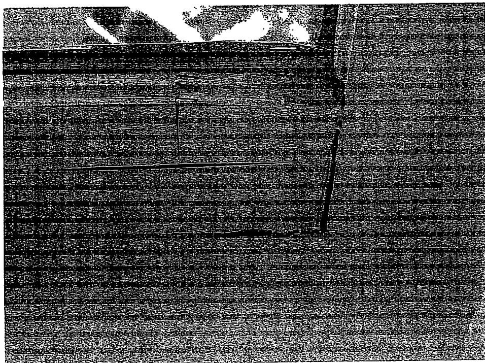
Figure 6 reveals the typical staining and deterioration observed on multiple windows from the interior of the gymnasium building. Note: this window, in unit 406, is identified as "new windows to match existing" on the architectural plans produced by Brock Green in 2000.
