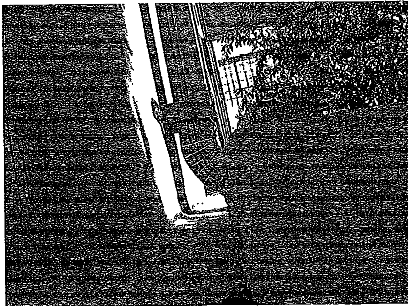
Figure 4: Close-up view showing the lack of wall through-wall flashing or weep screed visible at the stucco transition between the first and the second floor.
