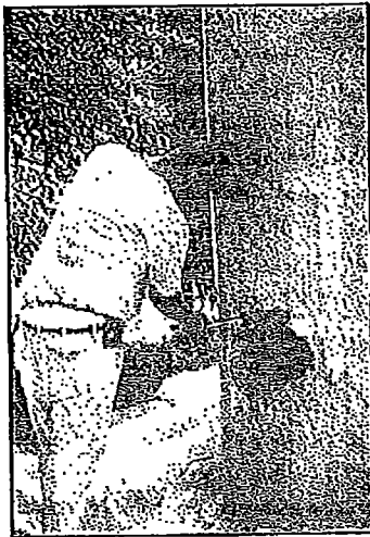
Fig. 4. Soft or crumbled plaster can usually be removed with a chisel or other hand tool. (69907)
