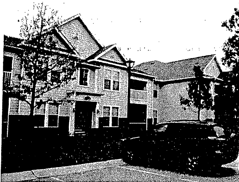
Front of Typical Unit
