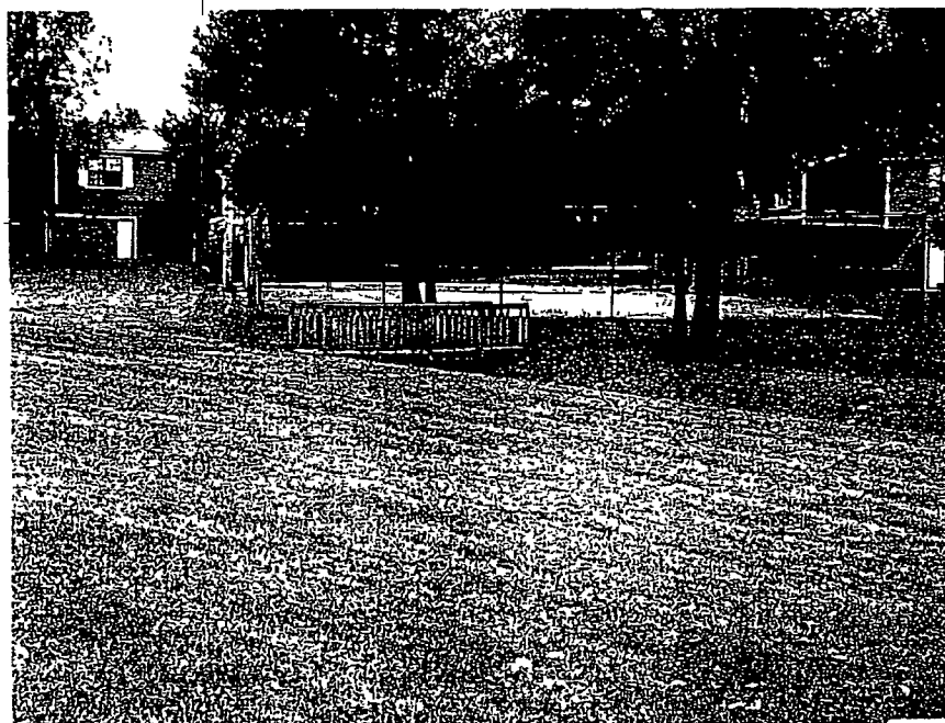
Photo 35 - Existing walk bridge
