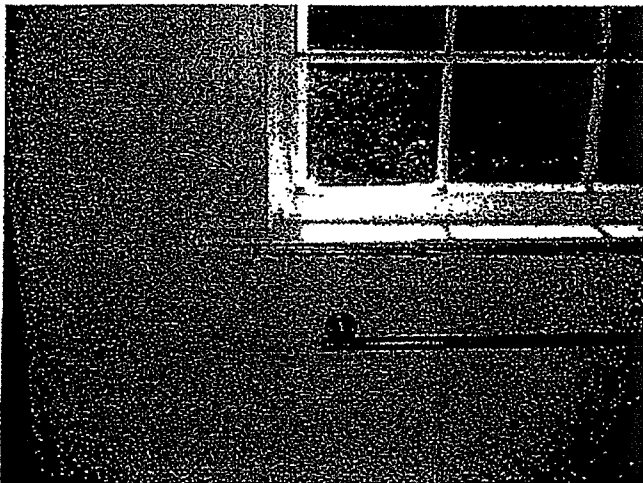
WINDOW TRIM MISSING. NEW WINDOW NOT INSTALLED
