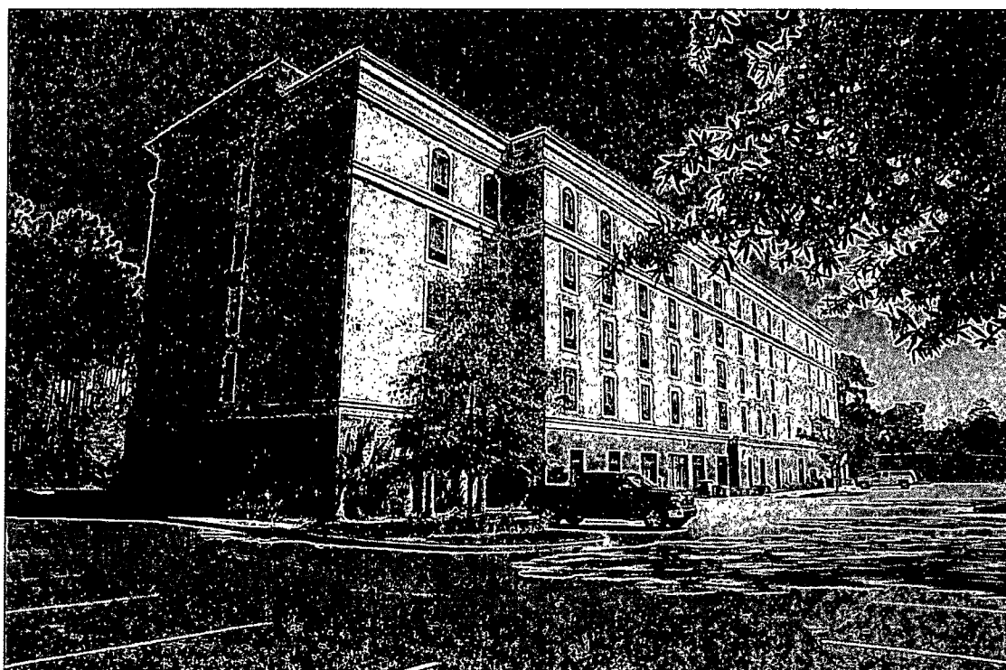
8. RIGHT SIDE & REAR OF SUBJECT (1576)
