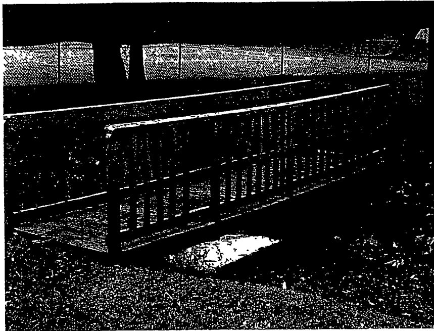
Photo 36 - Existing walk bridge
