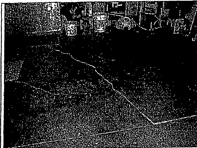
Cracking slab on grade at garage interior left side.
