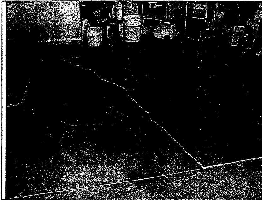
Cracking slab on grade at garage interior left side.
