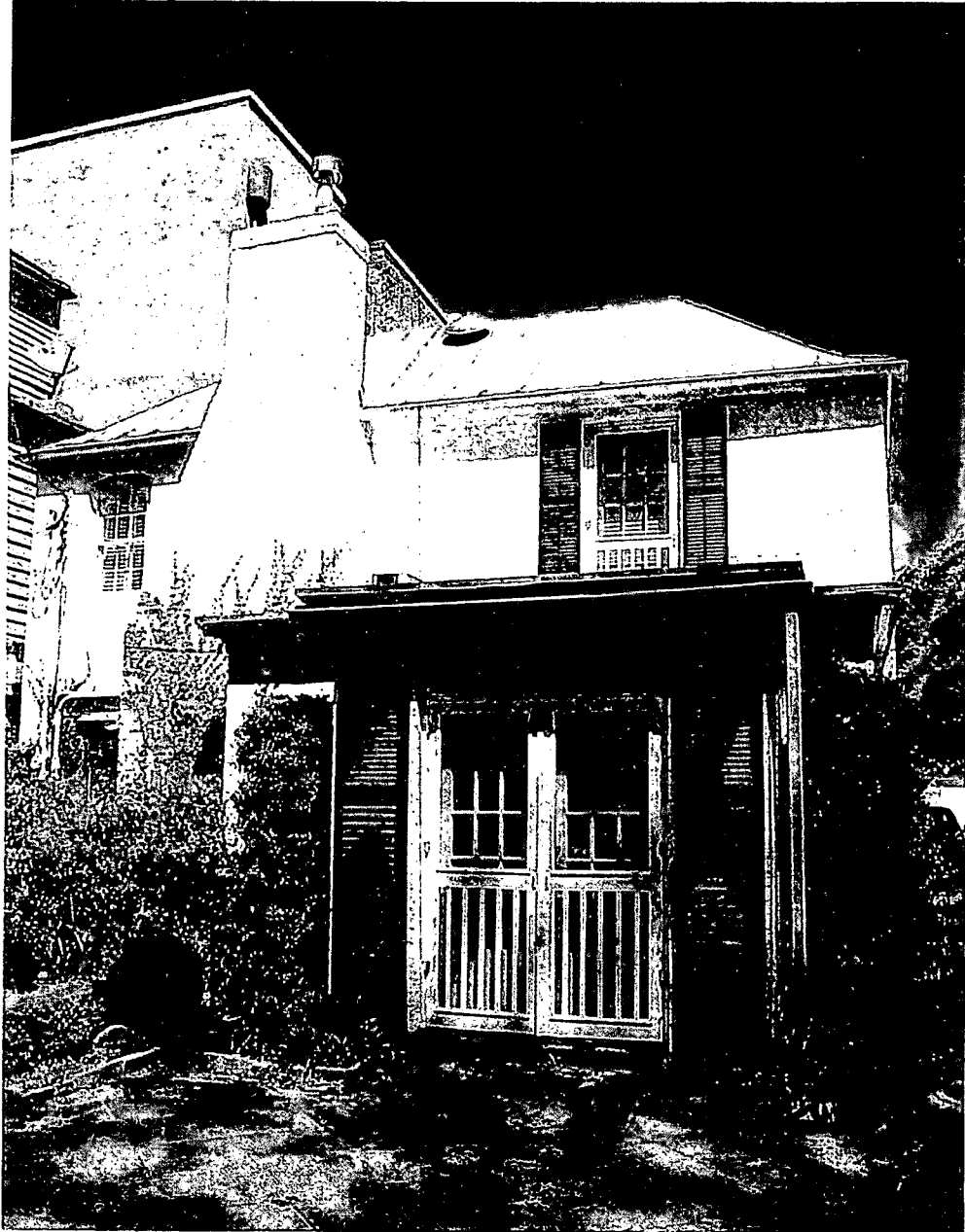
107 King Street. West Elevation ( Rear Elevation ). 1960's 1 Story Addition Approved By BAR for Demolition.
