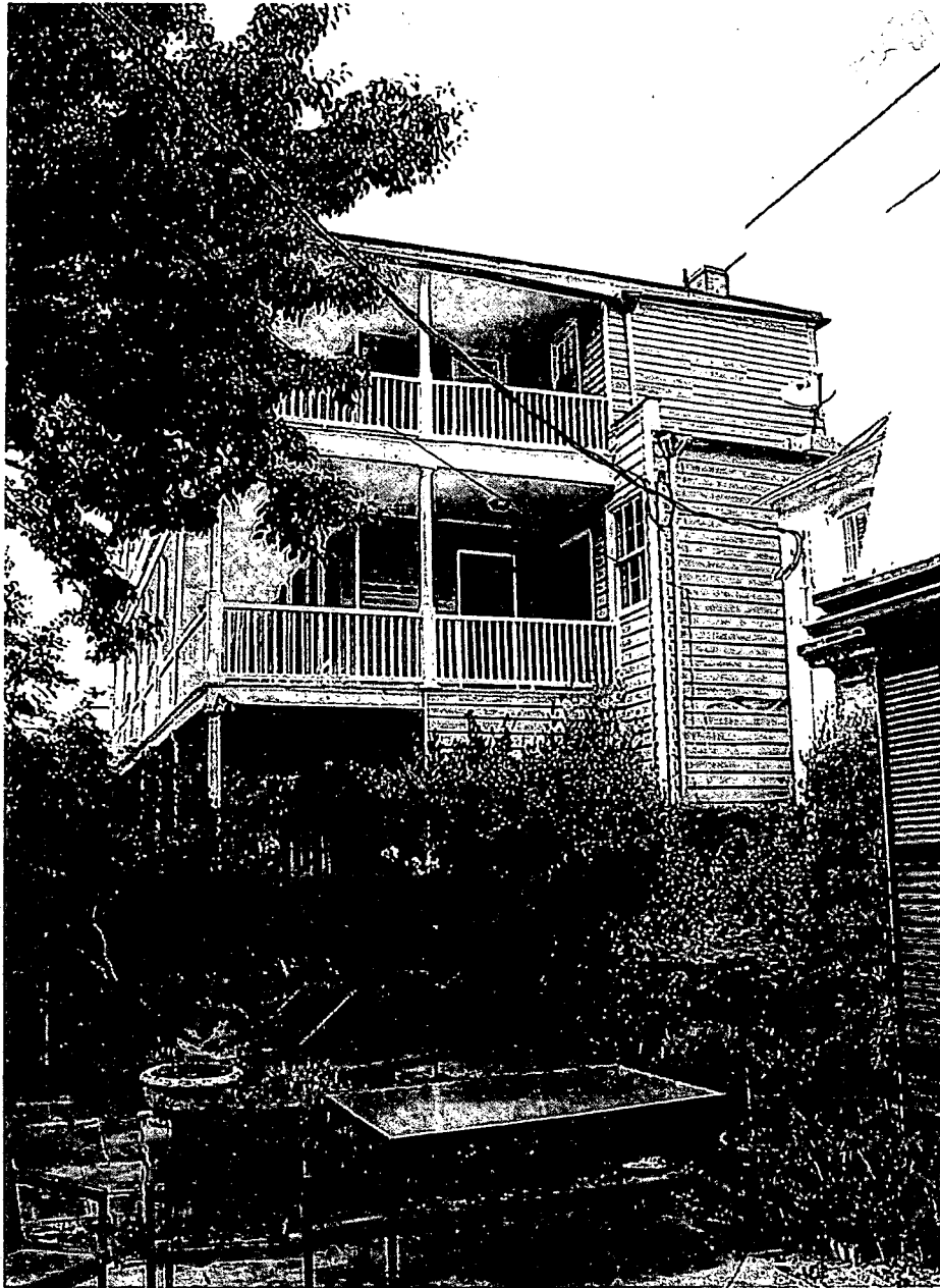
95 Broad Street. Rear Elevation. The North Elevation of 107 King Street Was Attached To 95 Broad Street ( As noted on Sanborn Maps ).
