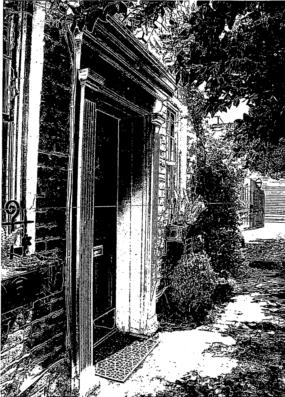
107 King Street. South Elevation Detail. Inappropriate Details such As Modern Ornate Door trim To be Removed and Replaced With A Simple Door Jamb as appropriate For A Kitchen House. Note : First Floor is on Grade.
