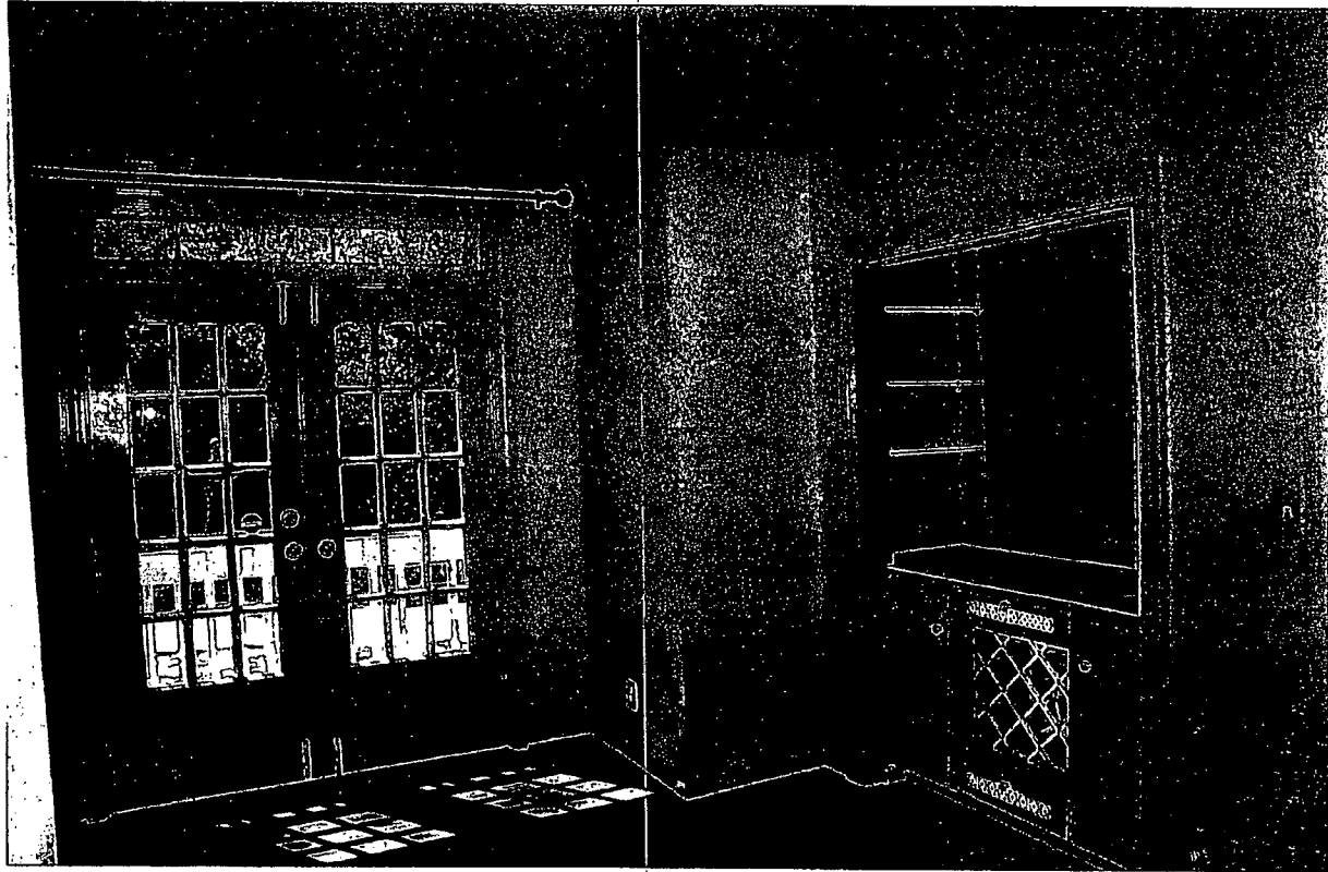
107 King Street - Interior of 1 Level Addition - Proposed Demolition
