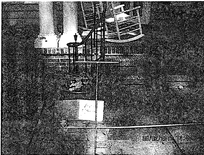
Photo 11: Front sidewalk and steps - Probe rod represents measured alignment of storm drain line.
