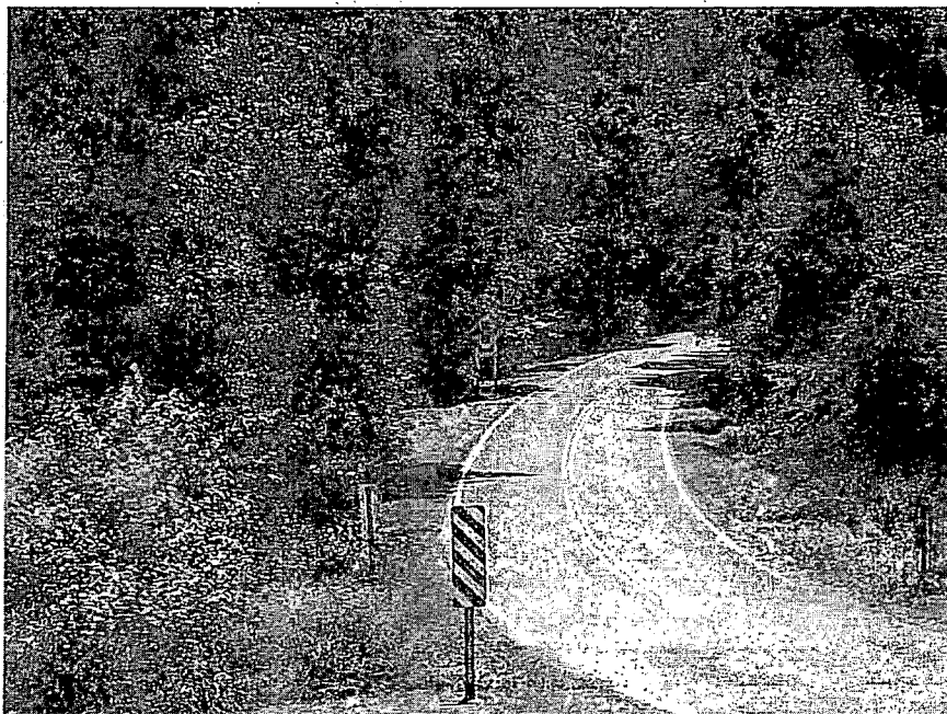
4. View looking south on Twin Lakes Road – subject on left (Taken 6/25/2014)
