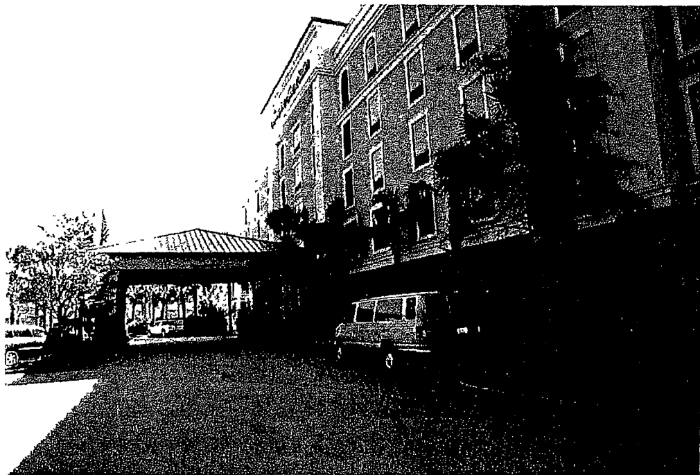
6. VIEW FROM RIGHT FRONT TO LEFT FRONT (1574)
