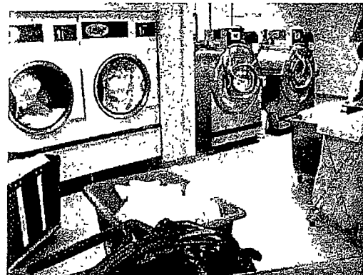
Hotel Laundry Room
