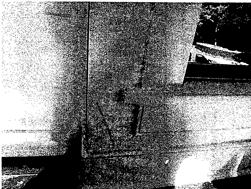
PHOTO 9A: View of water stains on interior drywall at underside of roof valley, South elevation. PHOTO 9B: View of moisture damaged interior drywall at breakfast room.
