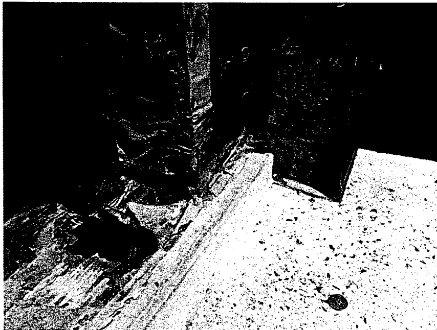
PHOTO 5A: View of French door pan flashing sloped to interior and back leg folded down. PHOTO 5B: View of rot damaged floor framing and decking at French door.
