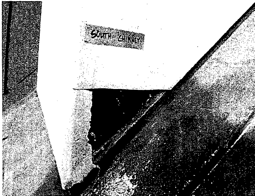
PHOTO 1A: View of South chimney test cut location and single layer of building felt. PHOTO 1B: View of incomplete building felt at roof-to-wall flashing.
