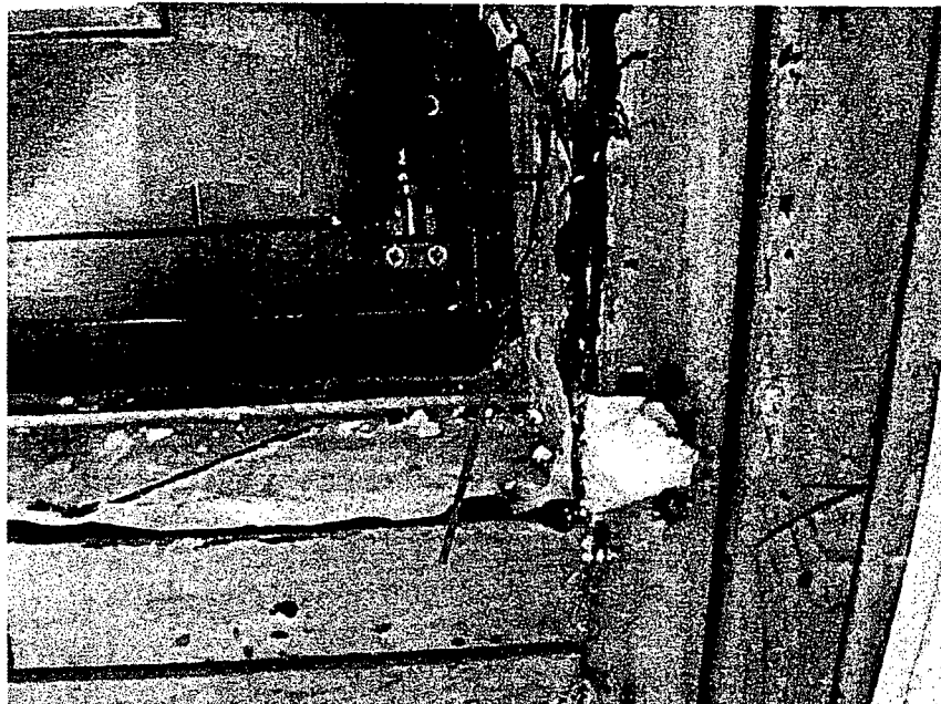
PHOTO 8A: View of gap in the sealant installation at master bedroom window, East elevation. PHOTO 8B: View of gap in the spray foam installation at perimeter of m. bedroom window.
