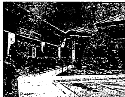
Midlands Technical College anchors the southern portion of the study area.
