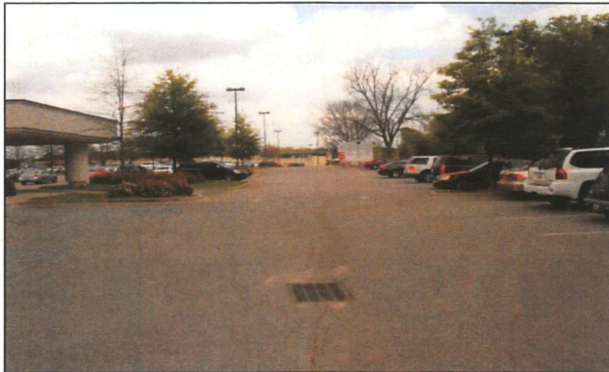
VIEW OF SURFACE PARKING AT FRONT OF SUBJECT MOB
