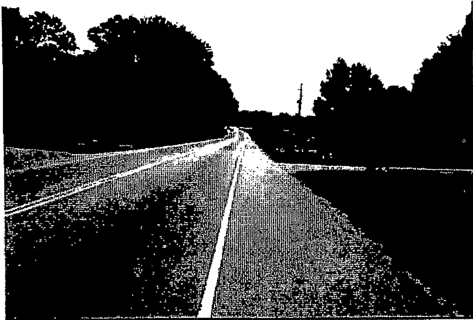
Photo looking north on US 29 toward the area of impact
