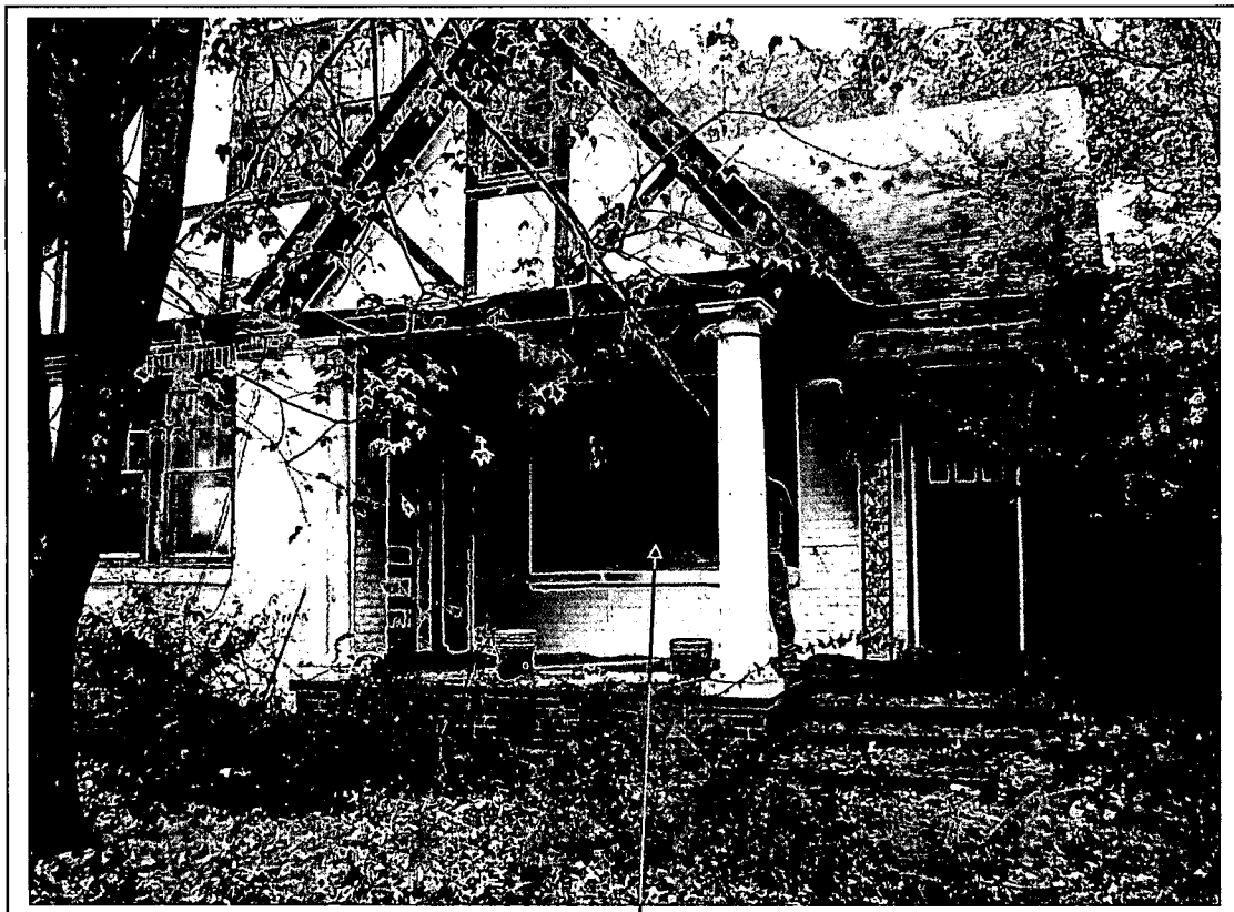
Windows removed without approval or permits.
