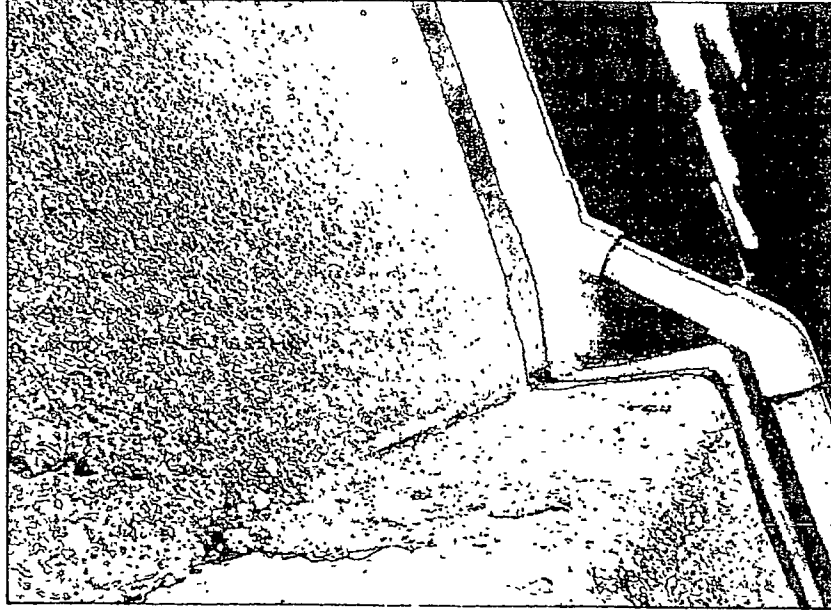
Figure 3: No base of wall through-wall flashing or weep holes were visible at the stucco transition between the first and the second floor.
