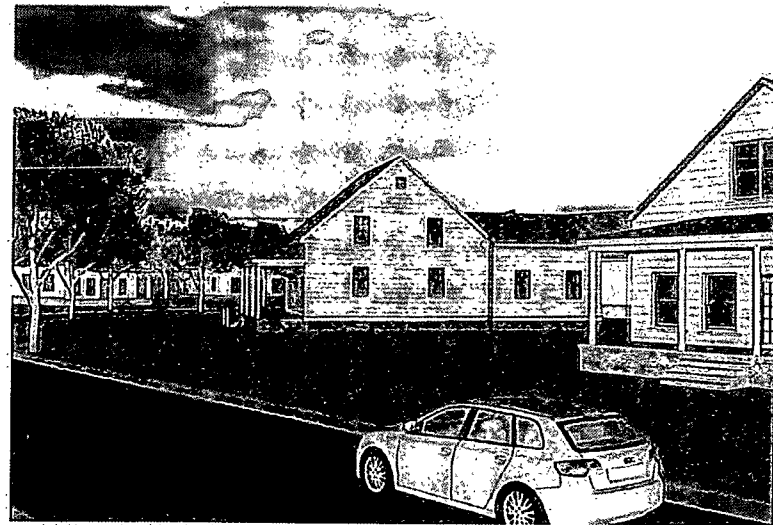
EXISTING CONDITIONS (IMAGE LOCATION 8)
