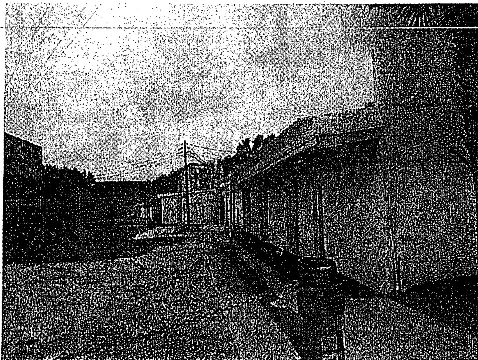
Southern side of building.
