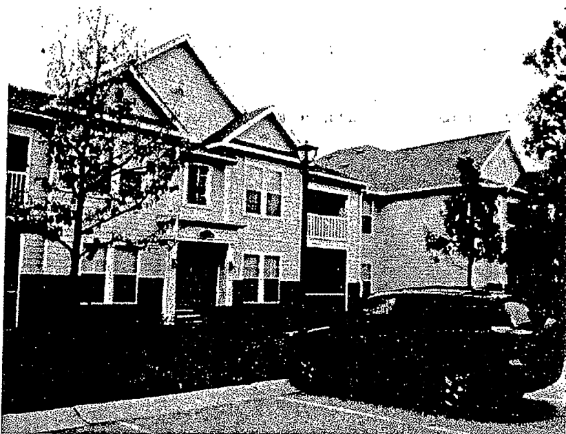
Front of Typical Unit
